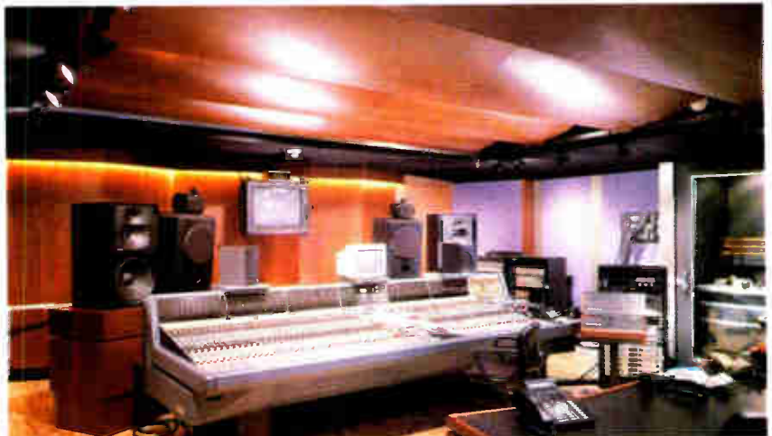
BMG Studios, New York City. Mix A opened April 1, 1994. Acoustical design is by Francis Daniel of Shen Milson & Wilke, and architecture is by Victor Schwartz of ARCooustics. Equipment includes a Neve VR60 console with Flying Faders, and Genelec 1038A tri-amped monitors. The rear wall has an all-glass, primitive root diffusor system, offering a view of the city and the Hudson.
