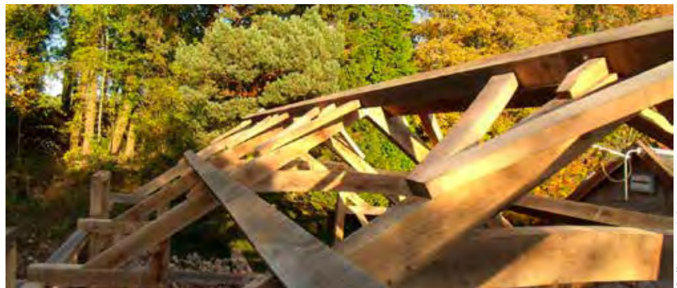
A home-grown oak frame under construction
