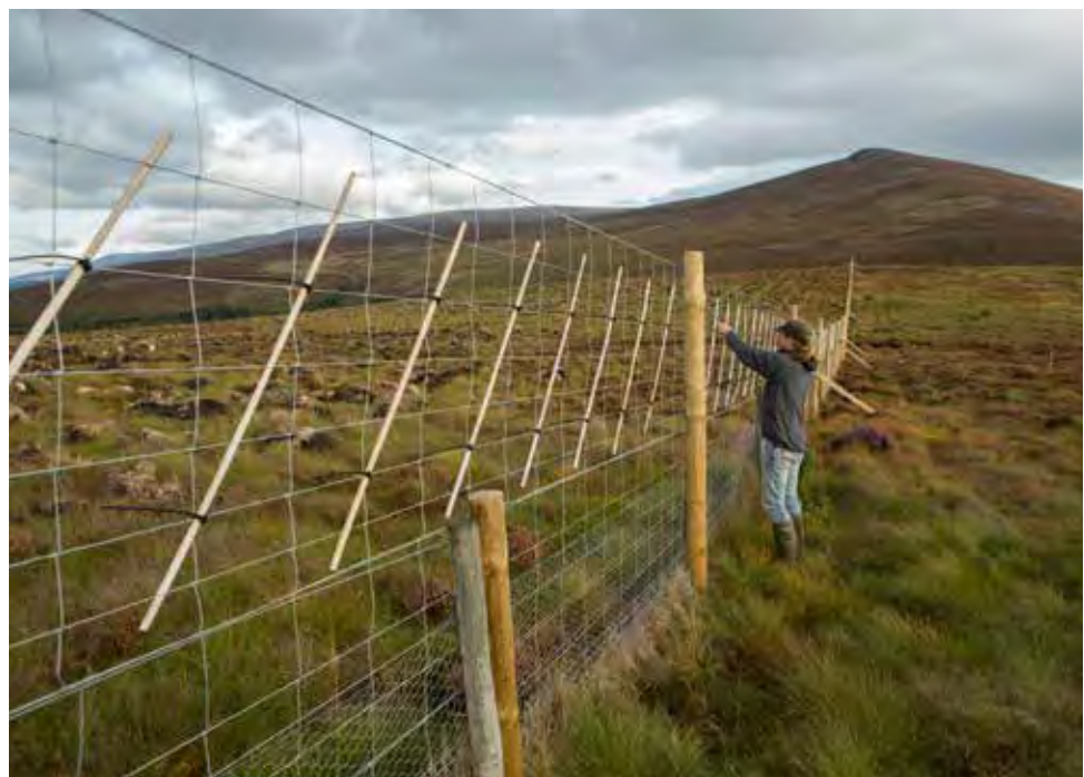
High specification deer and stock fencing with battens to increase visibility and reduce bird strike.
