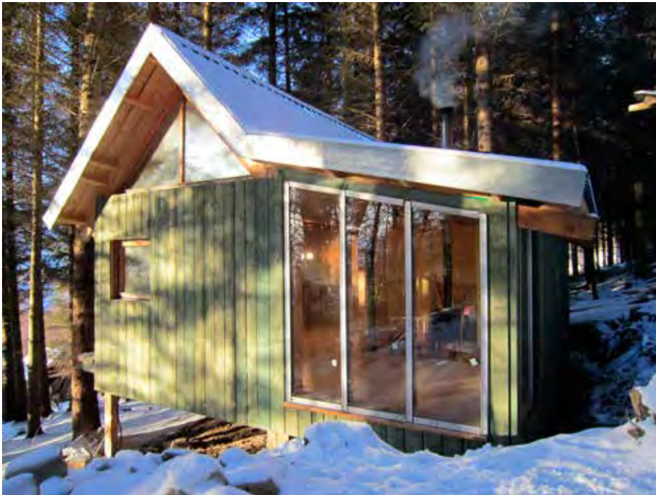
A 30 sqm hut clad in painted Sitka spruce in a Highland conifer plantation. Designed and built by North Woods.
