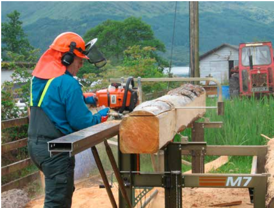
Logosol chainsaw mill: simple, inexpensive and effective giving high quality cut and plenty of exercise.
