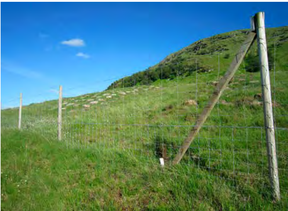
Deer fencing with two types of Rylock and top wire on newly planted site.
