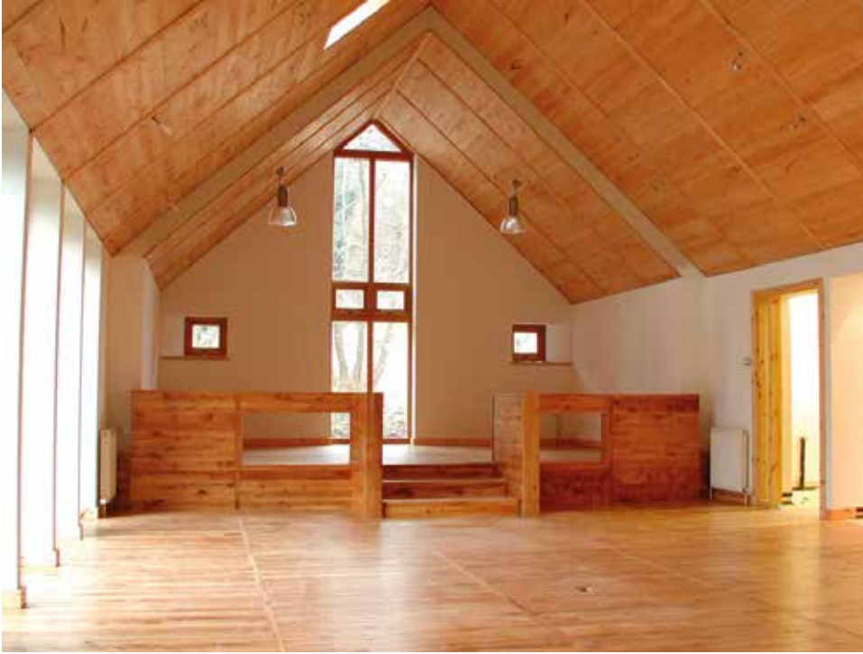
Scottish-grown birch ceiling and oak flooring in Glencoe visitor centre designed by Gaia Architects.
