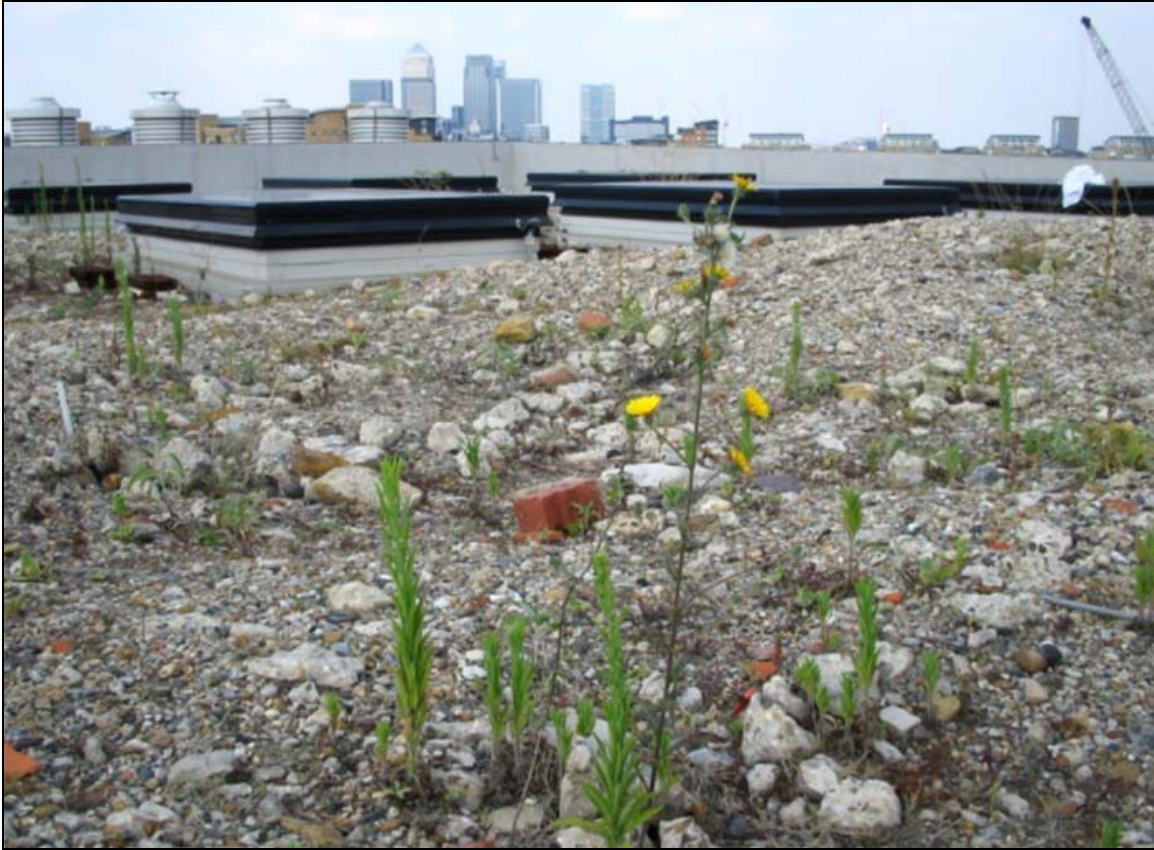
Figure 4. Black redstart roof three years after construction (photo by D. Gedge).
