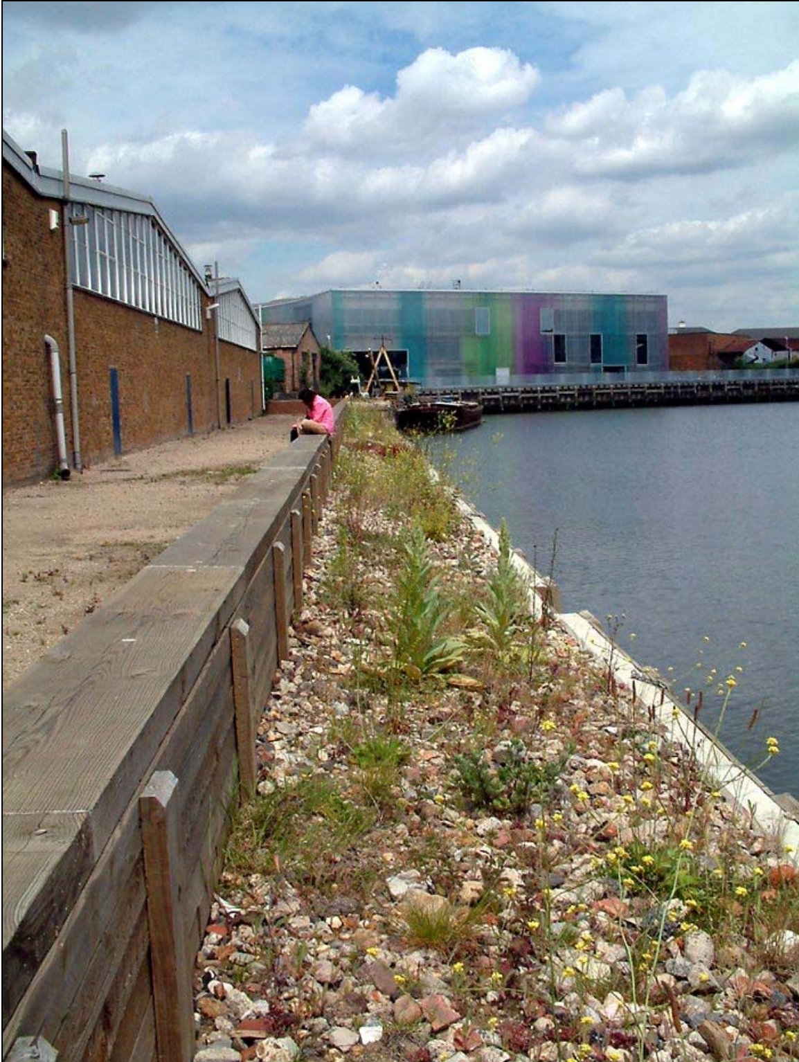
Figure 3: Sentinel, flood defence wall (brownfield site), Deptford, London.
