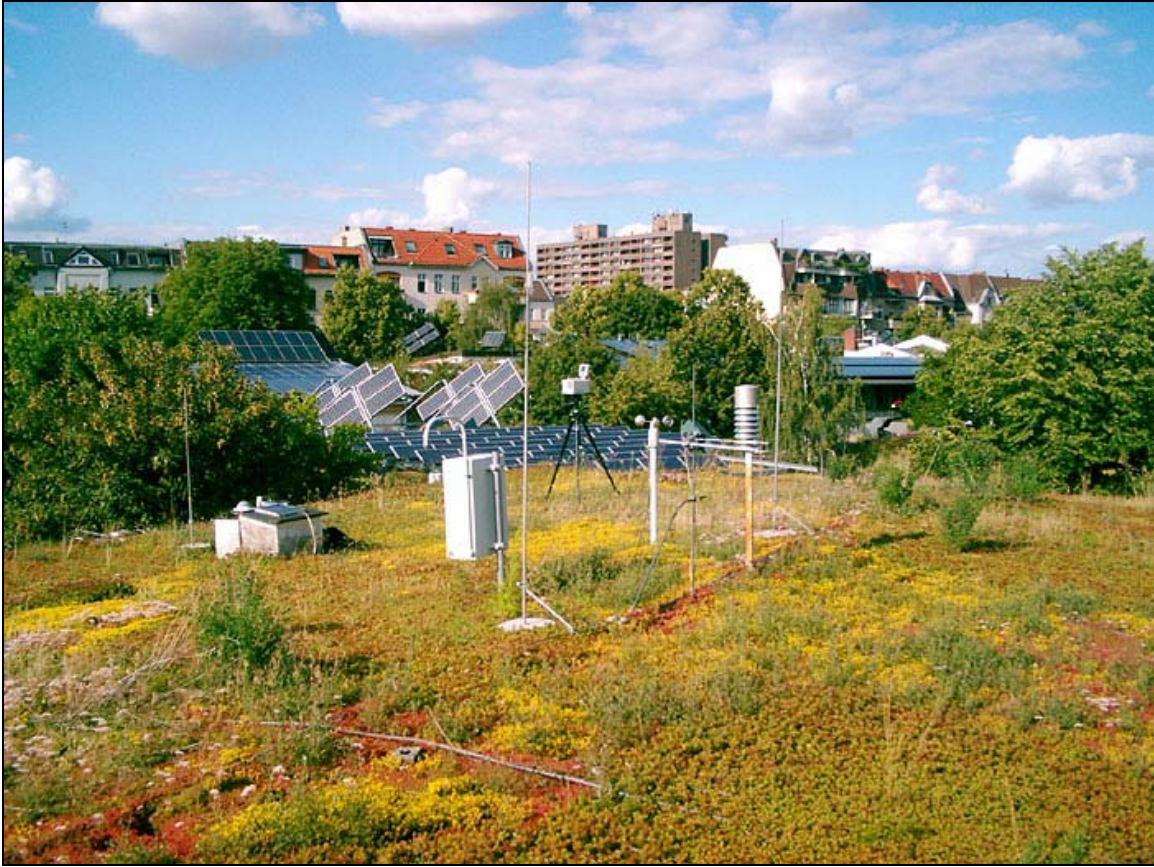
Figure 2b: The Ufa project EGRs in Berlin-Templehof: concert hall roof, with measurement equipment. Photovoltaic panels are visible on the adjacent green roof in the background.
