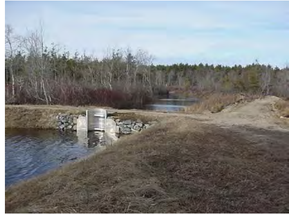
Fig 5. Flume with riprap. Outlet canal in back. Photo courtesy CCCGA.
