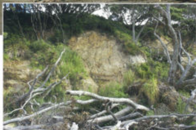
Pohutukawa-dominated bank undermined by high seas has collapsed on to the beach.
