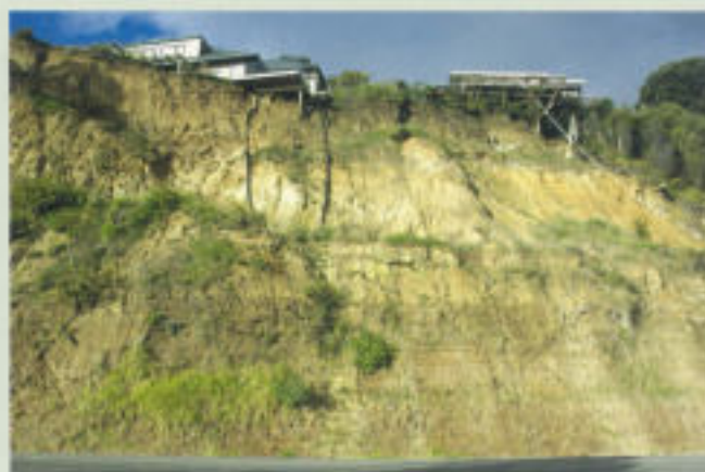
Cliff-top residential housing built as close as possible to the cliff edge becomes vulnerable as cliffs either naturally retreat or are subject to occasional slips that may be exacerbated by disturbance from the development
