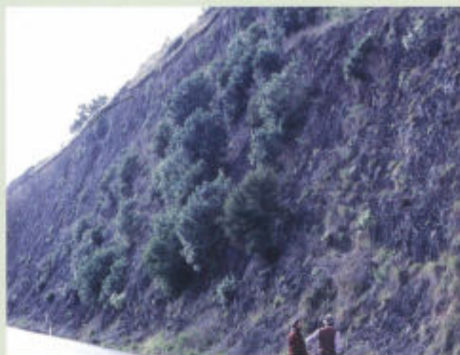
The exposed surfaces of cuttings and batters along coastal highways provide regeneration sites for pohutukawa where there is a local seed source.
