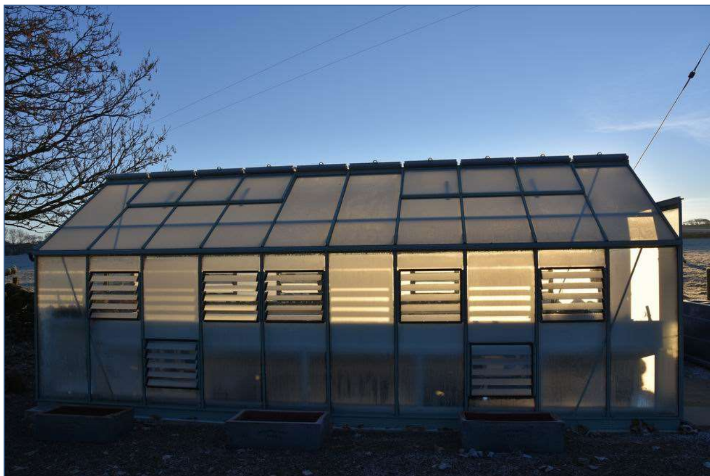
Early morning sun and condensation show up the vents on the house.
