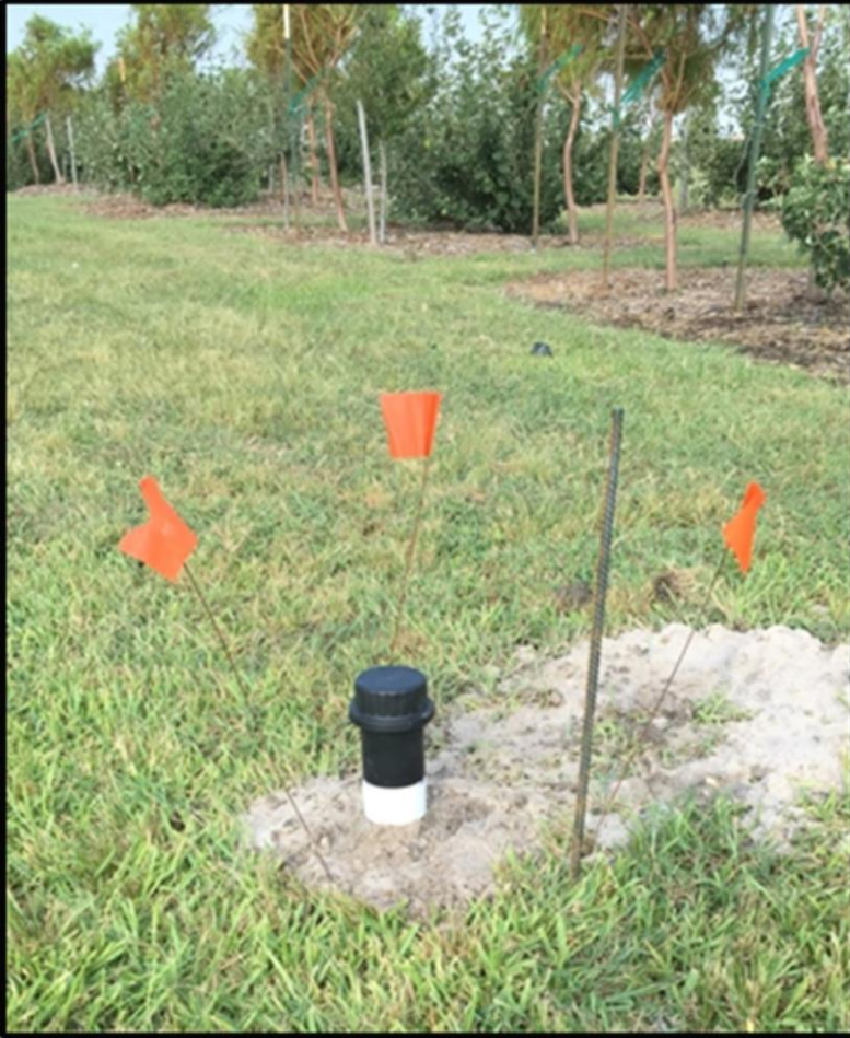
Image of typical installed piezometer at the Moody Gardens research site.
