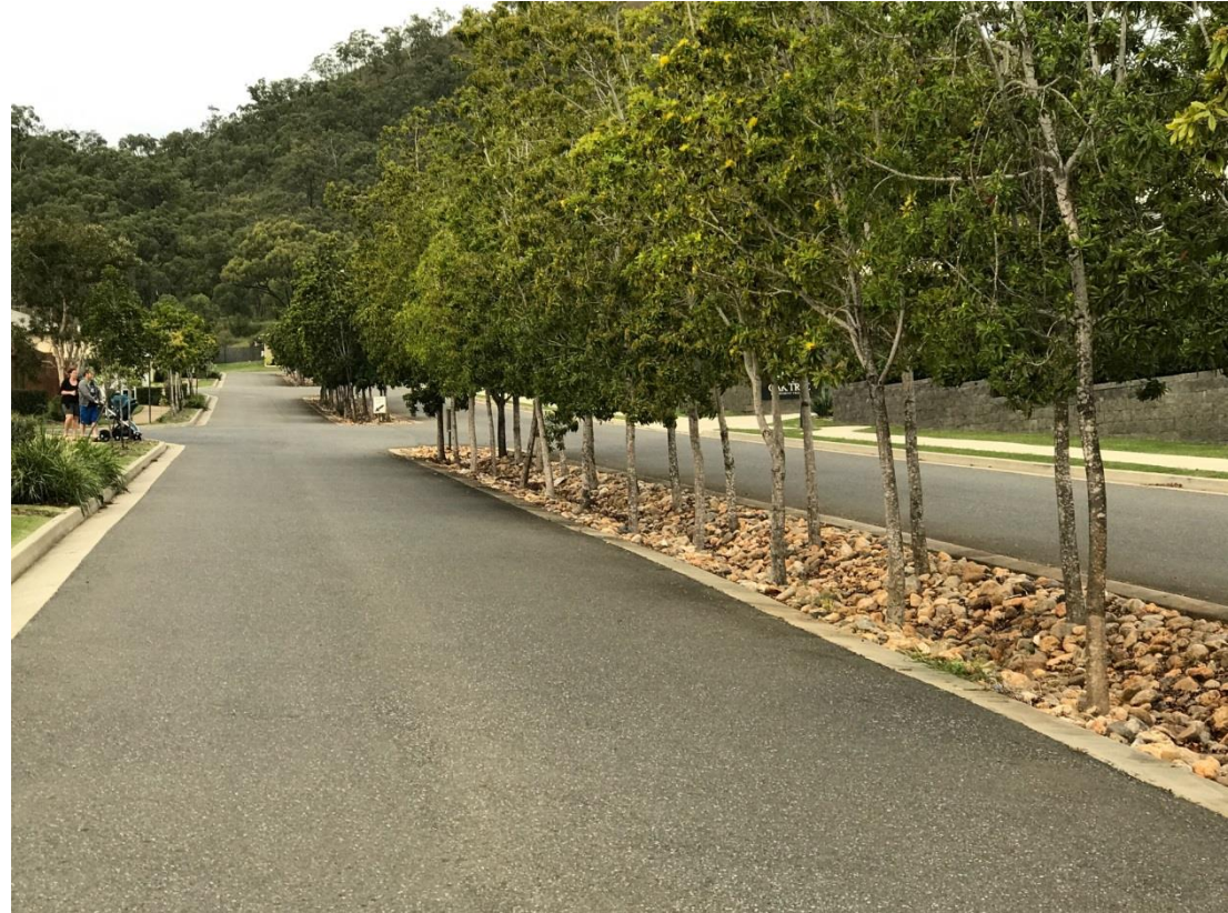
Creating leafy residential streetscapes that utilise water sensitive urban design
