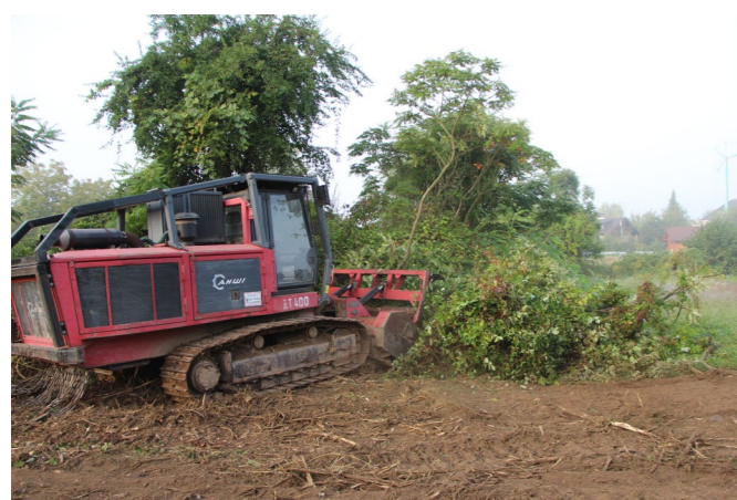
Figure 1: Cleaning the area with a mulcher
