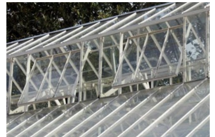
Figure 6: Automated windows
