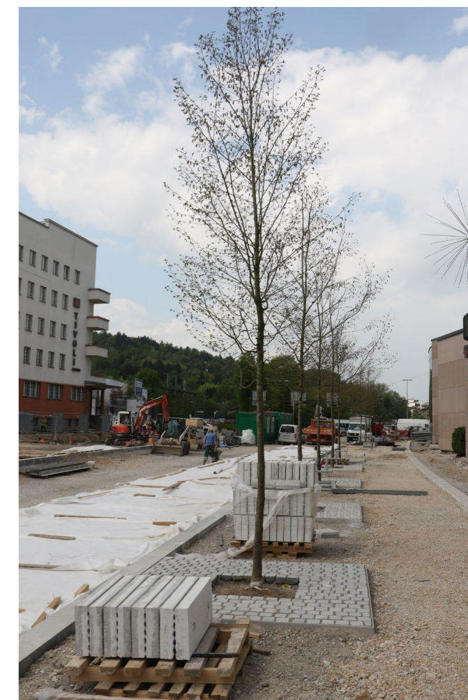
Figure 3: Last renovation of streets in Ljubljana in 2018
