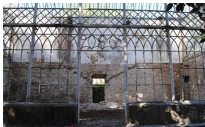
Figure 2: Restoration and rehabilitation
