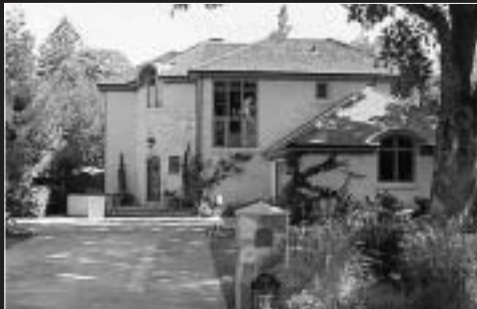
1014 Olive Street, Menlo Park (cross street: Santa Cruz Avenue) Offered at $2,695,000
