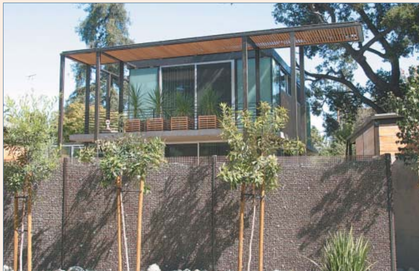
Joseph Bellomo's Palo Alto house, where he subtly integrated solar panels into the eave design, will be on tour Oct. 9.
