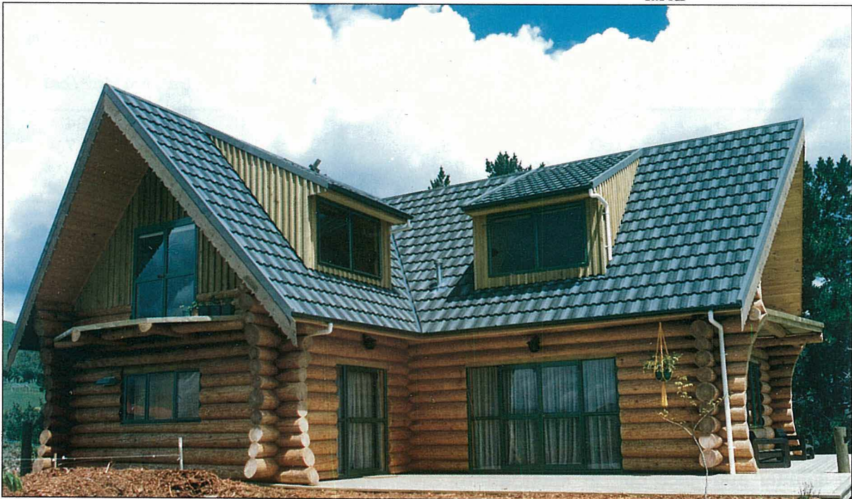
Fig. 16 - (below) Log house built in 1986 mainly of European larch
