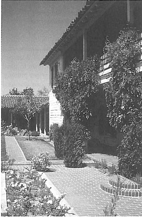
FIGURE 3. Lower terrace after treatment work. Certain courtyard features were rehabilitated based on changes in growing conditions. For example, original plant material was substituted with sun-tolerant plants based on the loss of the adjacent tree (the tree will be re-planted and original plants will be installed once the necessary growing conditions have been reestablished). Eugene O'Neill National Historic Site in Martinez, California. (NPS, c. 1988)
