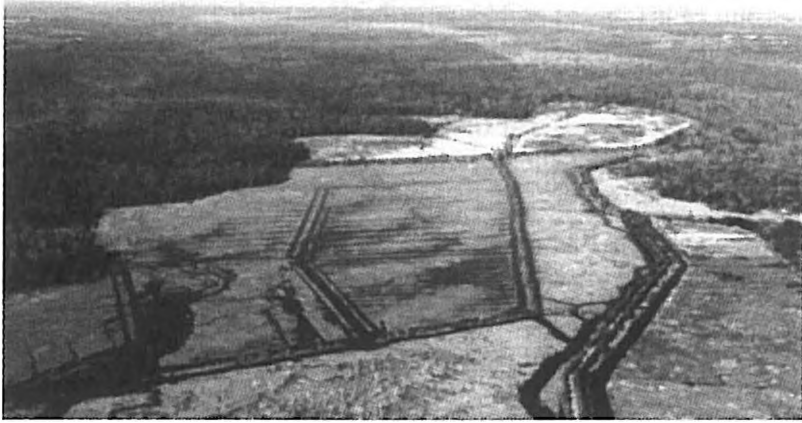
Tidal-influenced Former Rice Fields at Caw Caw Interpretive Park, Charleston County, South Carolina. These fields are now managed to promote wildlife habitat and provide seasonal viewing opportunities for future visitors to this regional park, now under construction.
