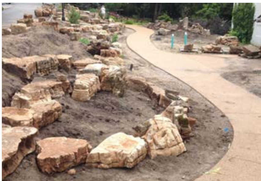
Looking east at the Bavarian Garden under construction.
