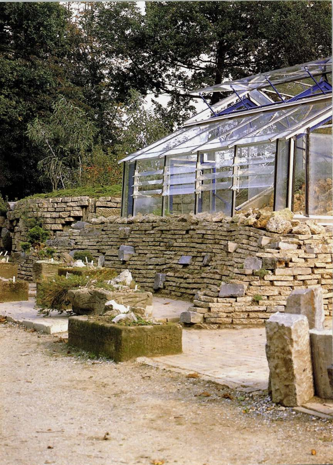
Alpine House at Utrecht Botanic Gardens, showing rock work with recycled materials (pp. 194-196)
