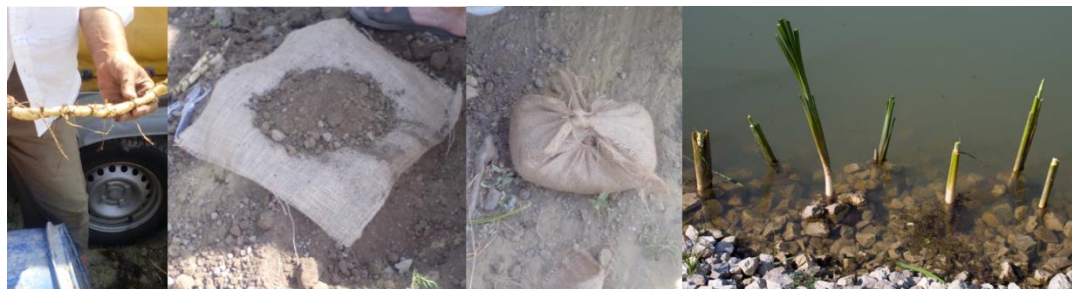
Fig. 2. The image series (from left to right) show the planting process and method of the riparian plants, in the case of rip-rapped bank surfaces
