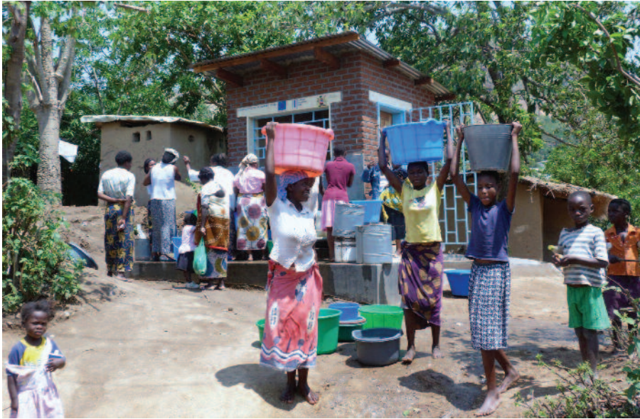
Water Kiosk constructed under the EU/EIB Project. Picture shows some of the beneficiaries from one of the water kiosks constructed under the Project. All Kiosks are bearing the logos of the EU, EIB and the Malawi Government to make sure that issues of visibility are well adhered to. (Picture courtesy EIB)
