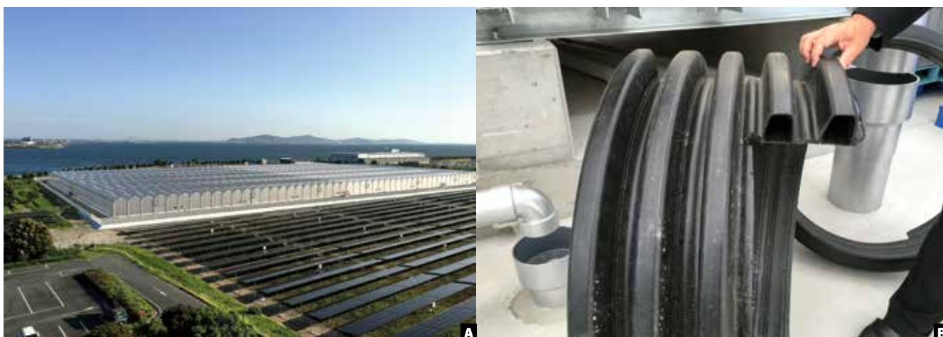
■ Figure 5. The base facilities in Aichi. A. Venlo type greenhouse. B. Heat is supplied from a sewerage facility.
