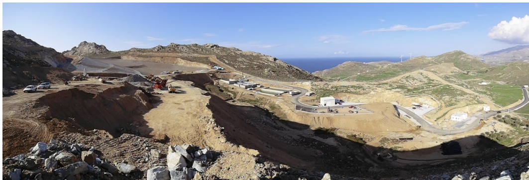
Fig. 7: Naxos Sanitary Landfill. Photo by Manolis Lykouropoulos.
