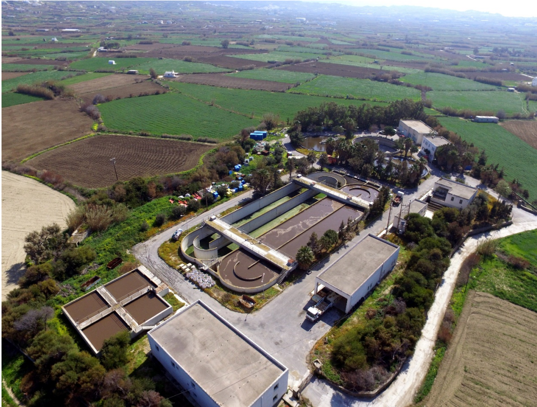
Fig. 11: Naxos Sewage Treatment and biological treatment station. Photo by Manolis Lykouropoulos.
