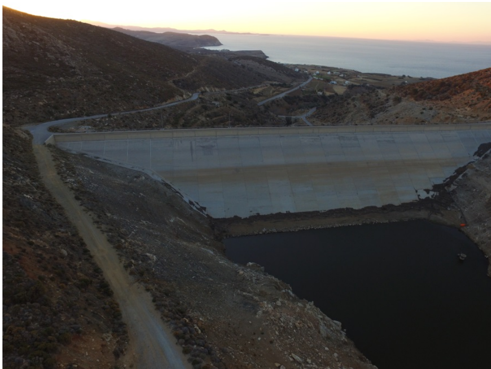
Fig. 36: View of the Faneromeni Dam, in the NW part of Naxos. Photo by Manolis Lykouropoulos.
