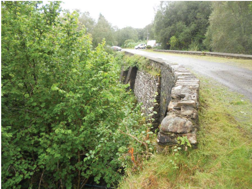
Image 13.2 Road bridge on the Allt Torr nan Daoine
