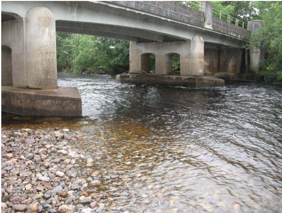
Image 13.11 River Carron at A890 road crossing
