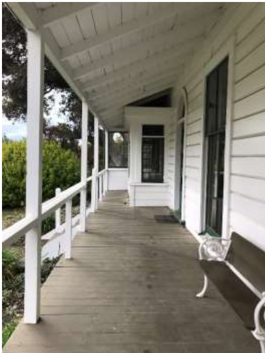
Verandah looking east
