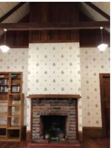
Fireplace in west bedroom
