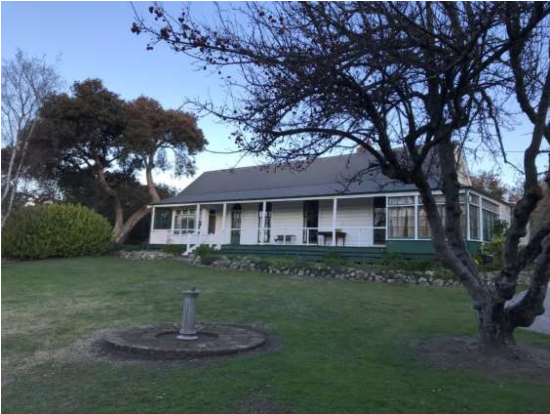
Figure 13: View to the north side of Keirunga Homestead. Matthews & Matthews Architects Ltd, August 2020.
