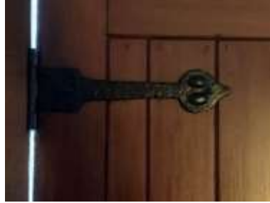
Wrought iron hinge rear door
