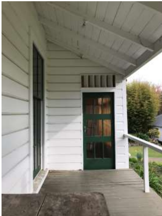
Verandah looking west
