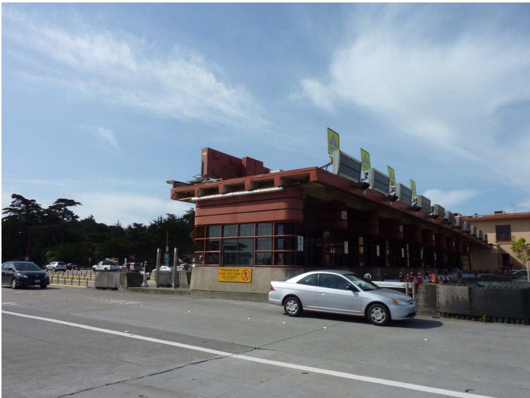
Photo 14: Toll Plaza looking West
