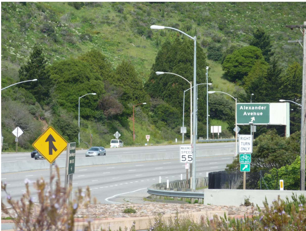
Photo 2: Permanent median strip North of Bridge
