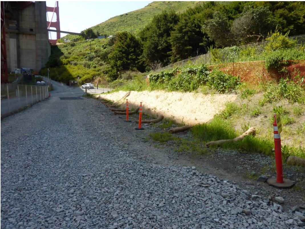
Photo 6: North side of Staging Area 2 looking South
