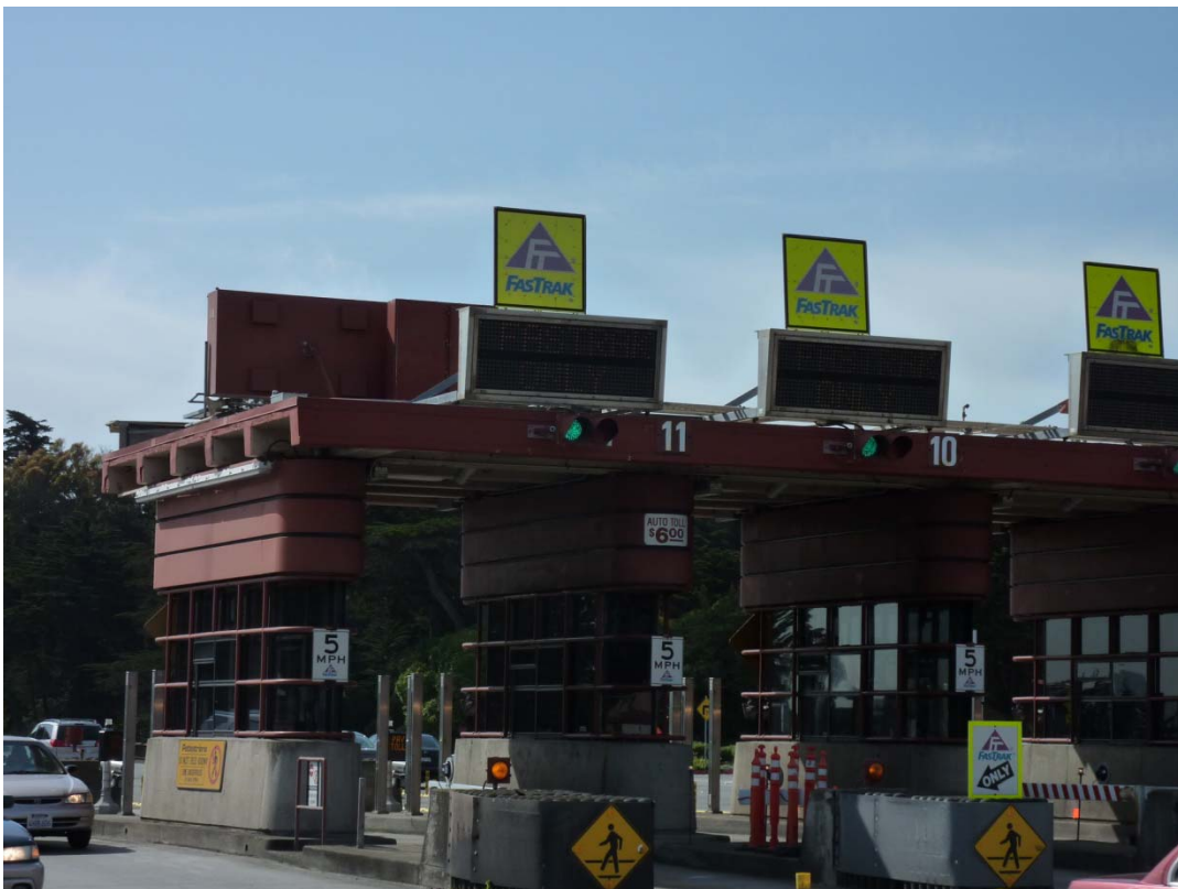
Photo 12: East end of Toll Plaza looking South
