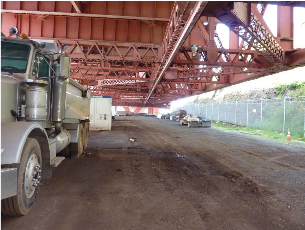
Photo 9: Staging Area 4 looking South; located below North end of Bridge
