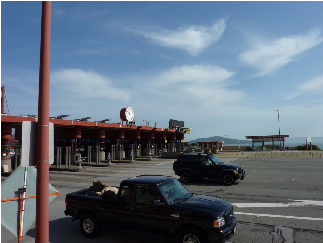
Photo 13: Toll Plaza looking East
