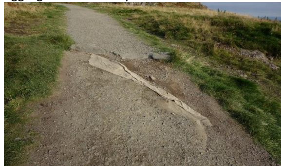
Fig 7. Path surface washed away to reveal underlying membrane.
