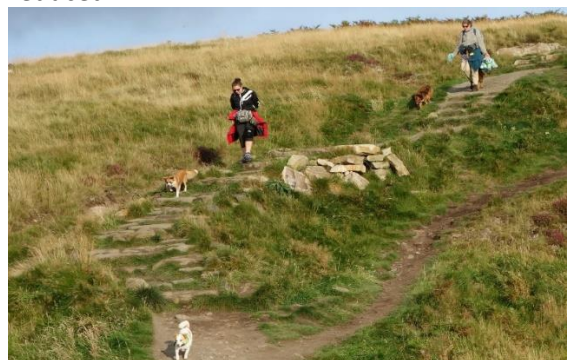
Fig 4. Dog walkers on a stretch of stone pitching on a steeper section. Note biker's path to right
