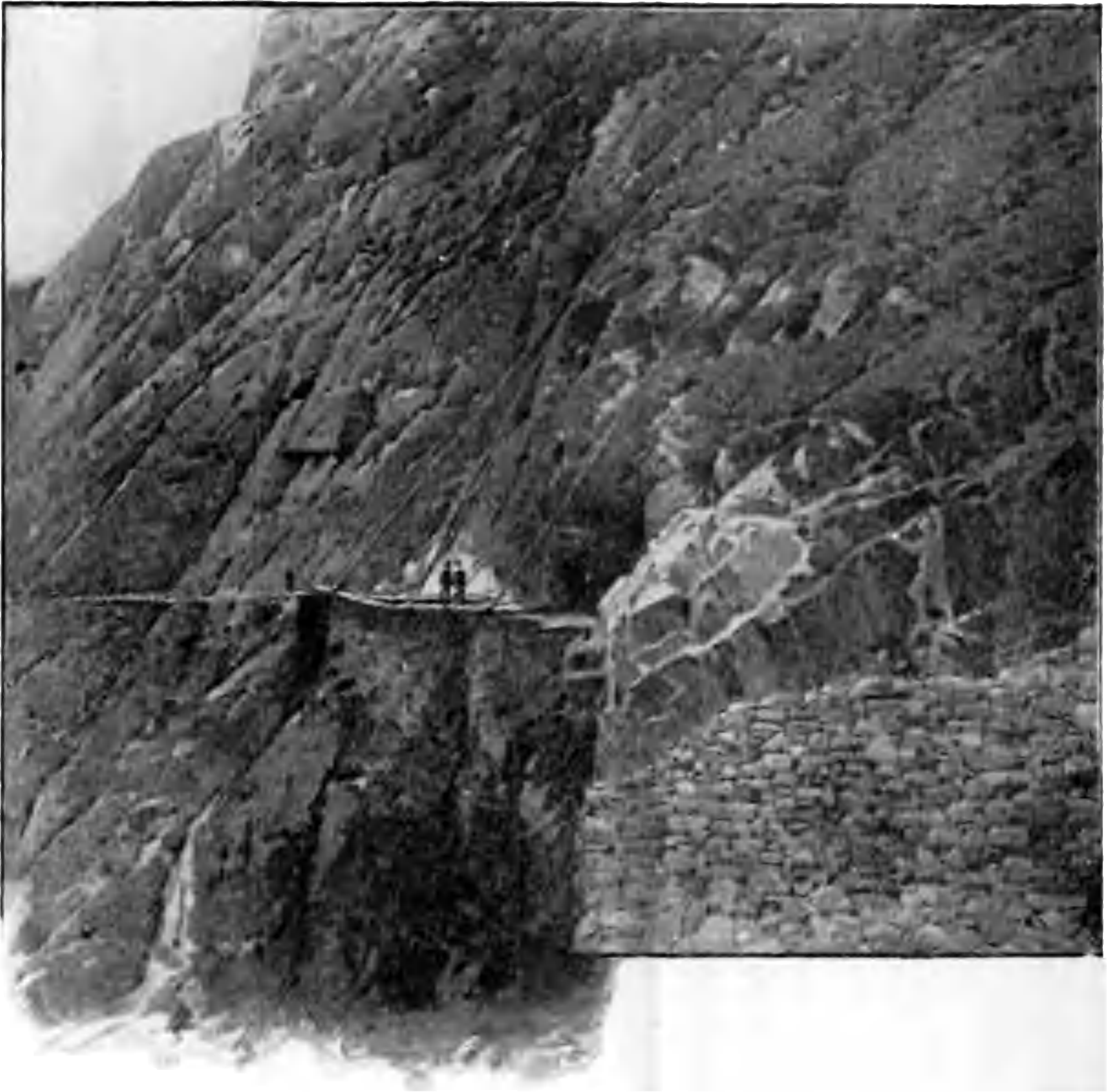
A SHAKY PASSAGE ON THE NERPANI ROAD
