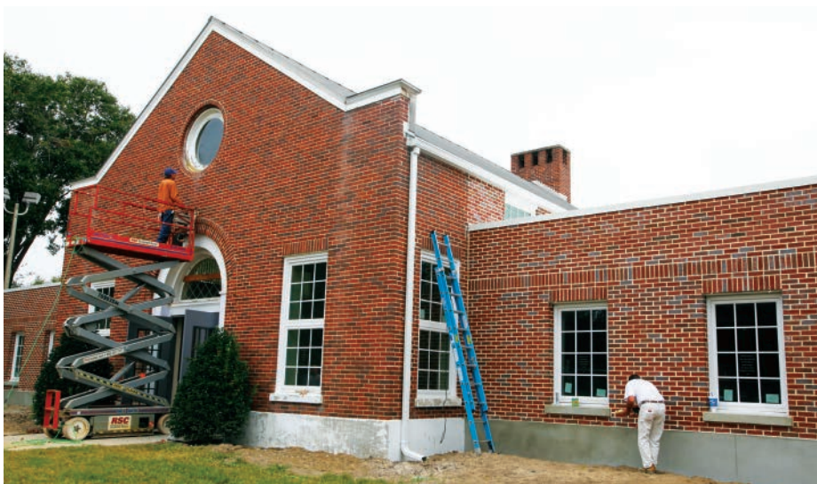
The Fannin Campus Ministries Center nears completion.
