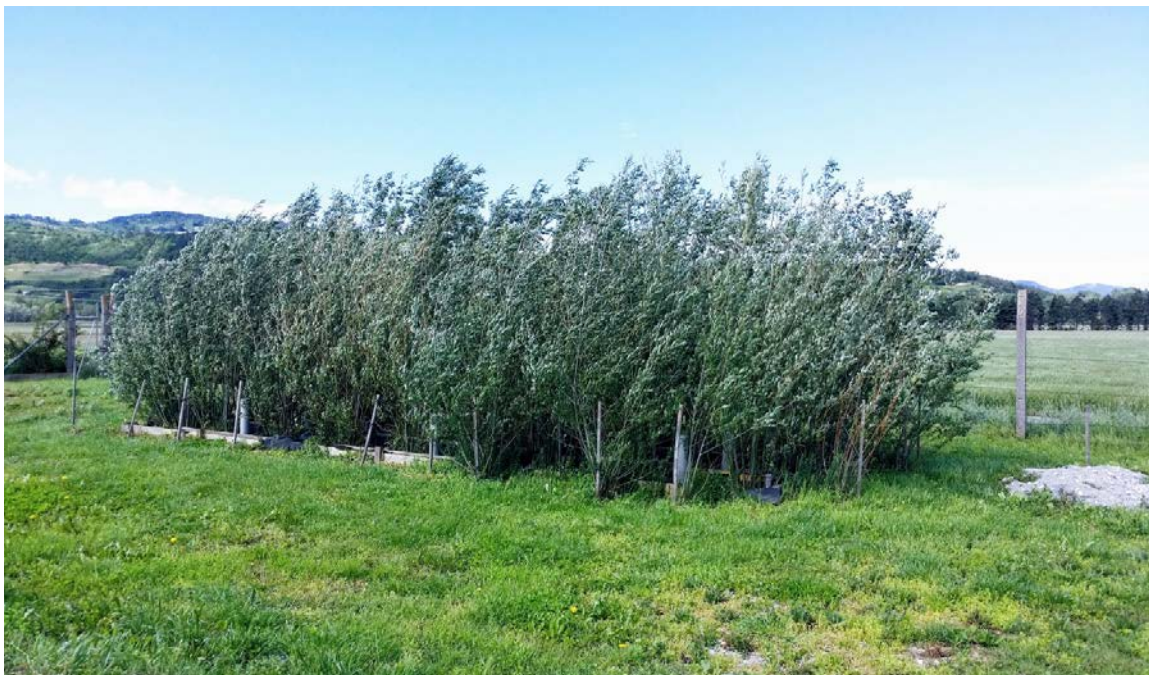
Figure 2: Pilot evapotranspirative willow system for treatment of municipal wastewater in Ajdovščina, Slovenia (Photo: Darja Istenic)
