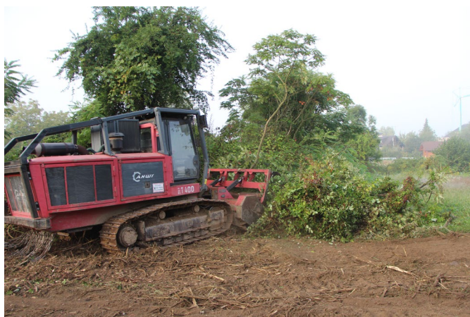
Figure 1: Cleaning the area with a mulcher
