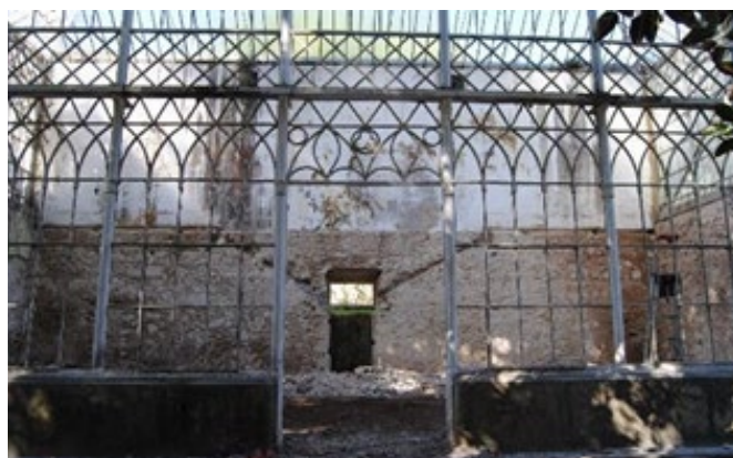
Figure 2: Restoration and rehabilitation
