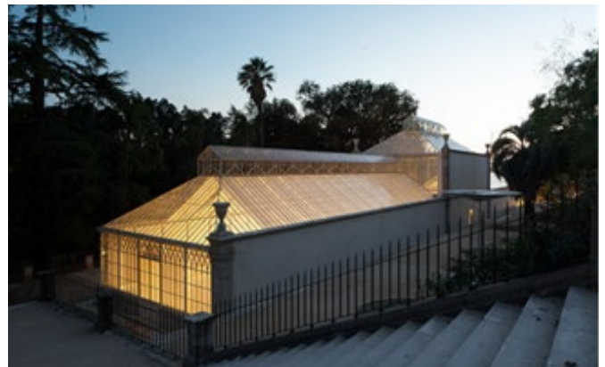
Figure 12: The surrounding area of the greenhouse was also rehabilitated
