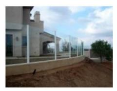
Figure 6. Example of Heat Deflecting Wall
