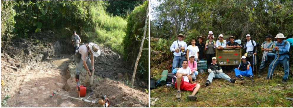
Left: Recovery and clearing of the Lengerke Trail with volunteers of YARÉ II in Zapatoca. Right: Ecoroute tour Lengerke Road with community in San Vicente de Chucurí and information billboards. © D. Villanueva/YARÉ.
