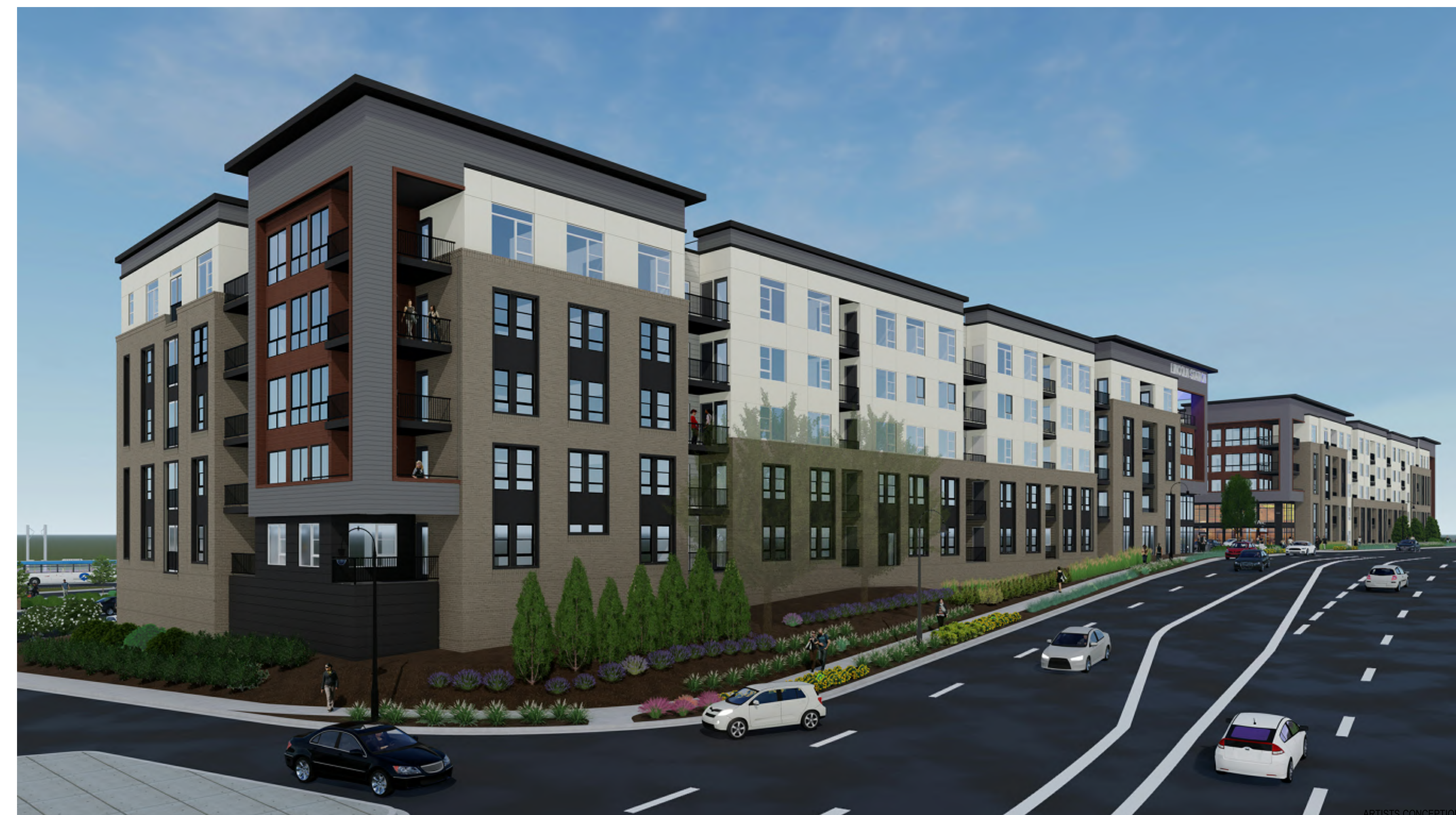
PARK MEADOWS DRIVE NORTHWEST CORNER
