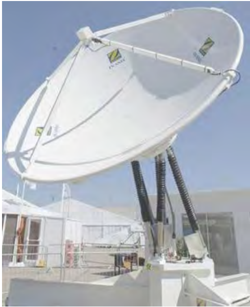
Figure 2-7: SANSА (1,2,3) This is a typical 6m antenna with a height of up to 12m.
