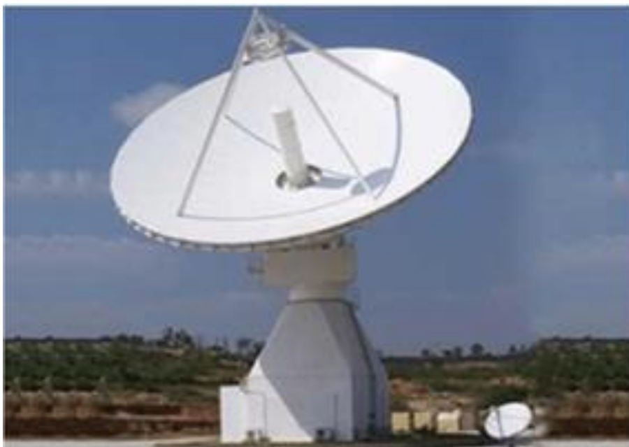
Figure 2-7: LGS18, Ka Antenna, 18m wide dish, 30m height.
