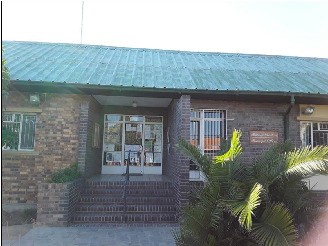
Laingsburg Municipal Office
