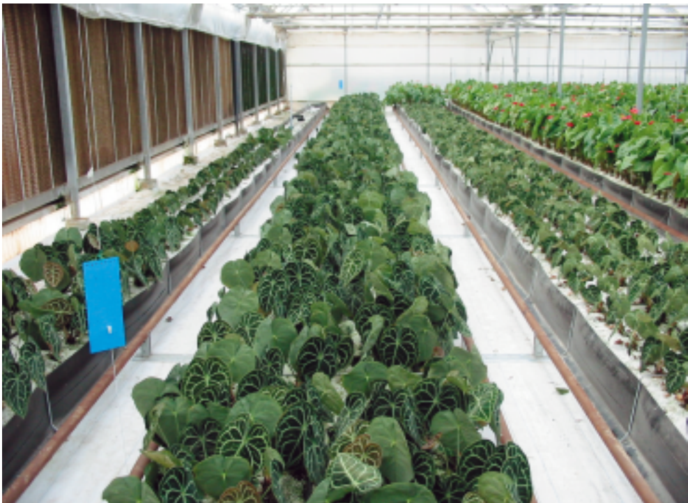
Paneles interiores de cooling system.
