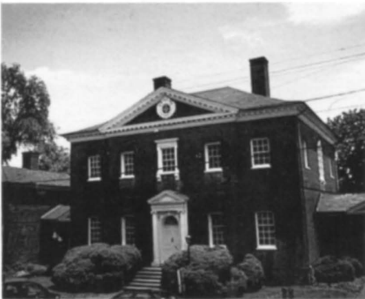
Hammond-Harwood House with massive boxwood at the entrance. (Photo: Scot Butler)
