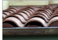
Figure 6. Birdstops prevent debris from accumulating under tiles. Photo: Stephen L. Quarles
