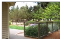
Figure 50. Wooden framing with wire mesh (Division of Agriculture and Natural Resources)
