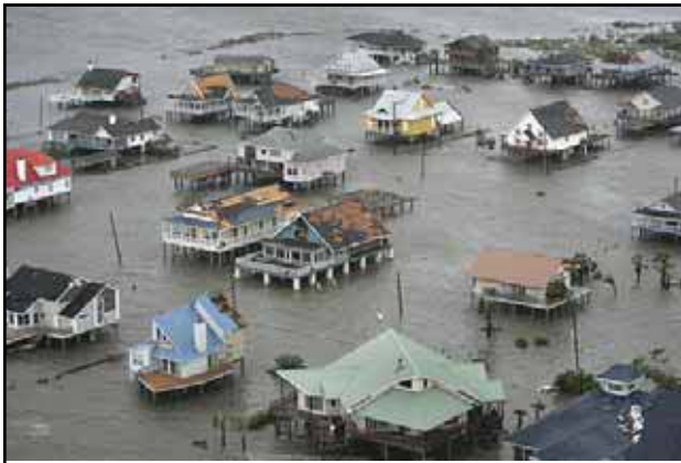
Elevated homes in Sweet Lake, LA (near Lake Charles) after Hurricane Rita (09/24/05).
