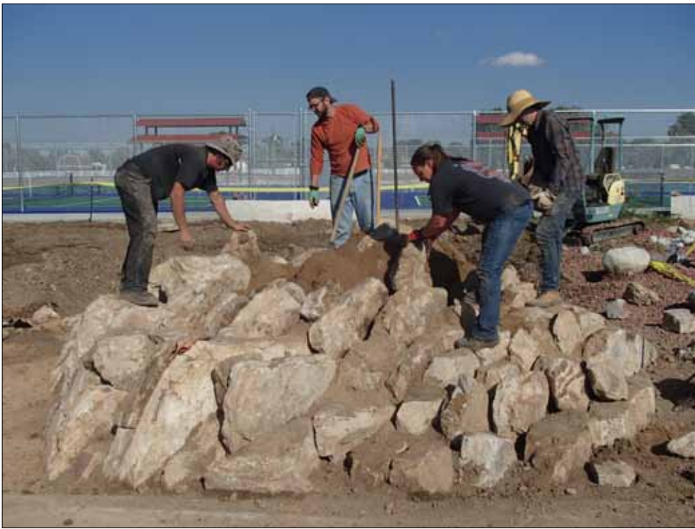
First mound (#5) under construction
