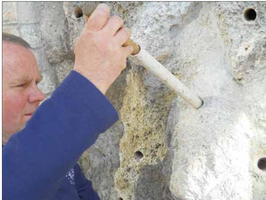
Ramming home the compost mix
