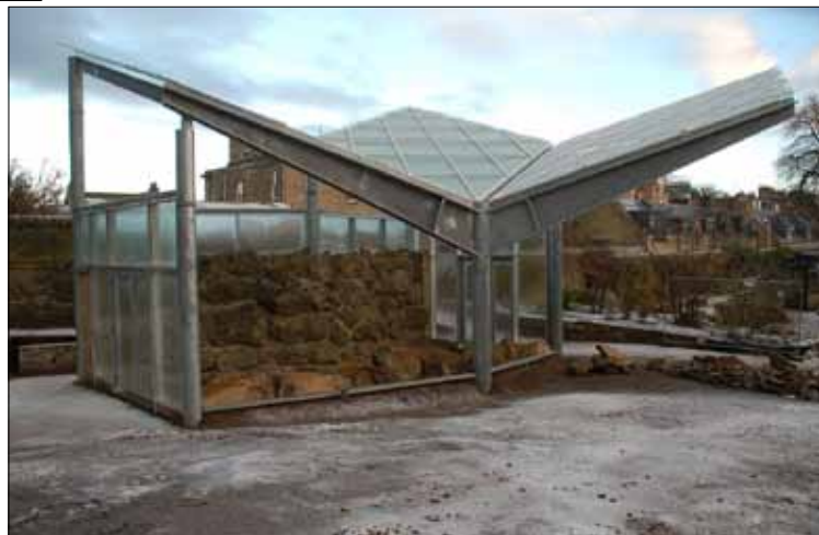
The tufa wall in place in December 2012
