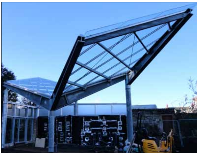
Back Wall in place in November
