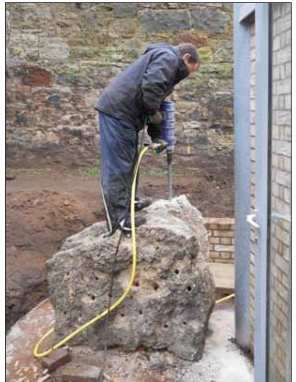
Drilling one of the 600 holes
