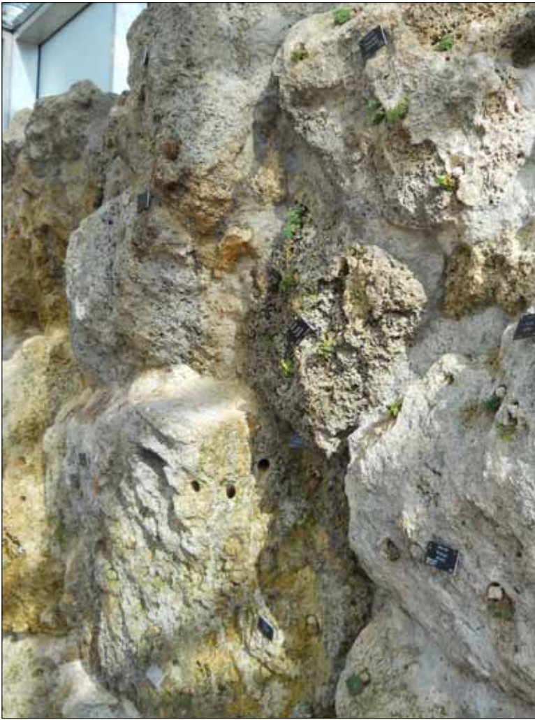
Tufa wall close up
