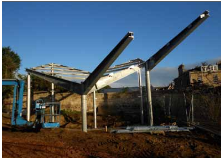
Steel and glass goes up in September
