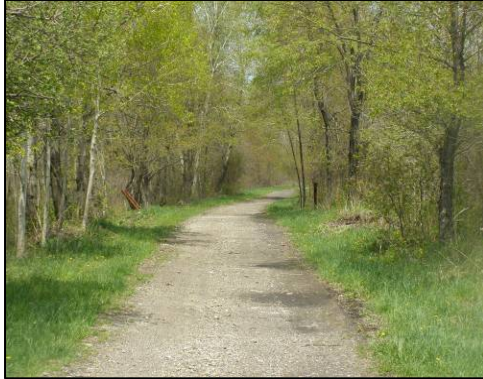
A section of the Corry Junction Greenway Trail
