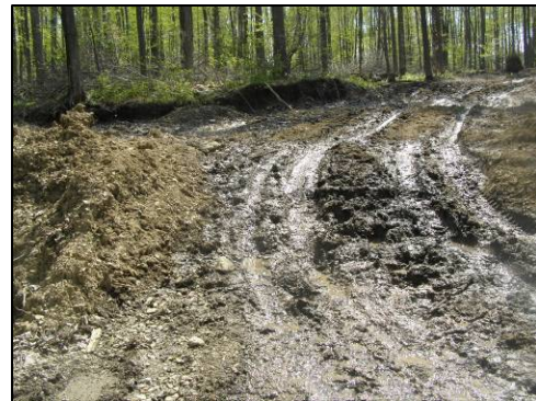
Runoff from a logging road
