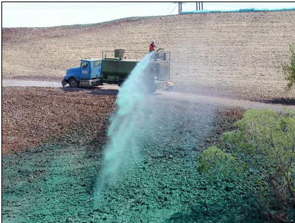
Figure 6. Flexterra application on a hillslope at the Site.
