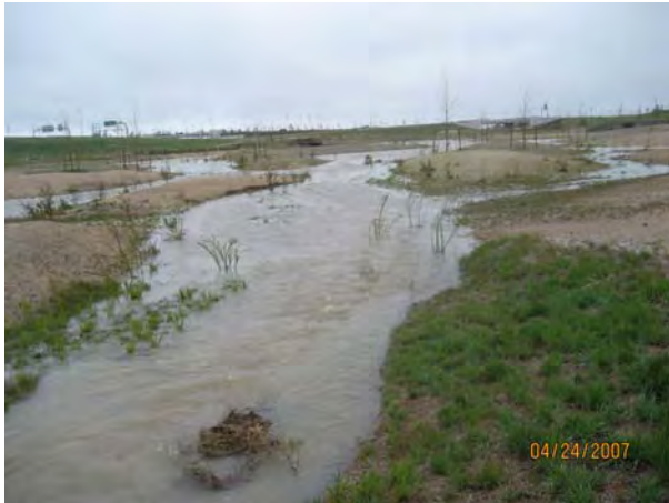
Figure 15 - View looking north at cut-off wall between Cells 2 and 3
