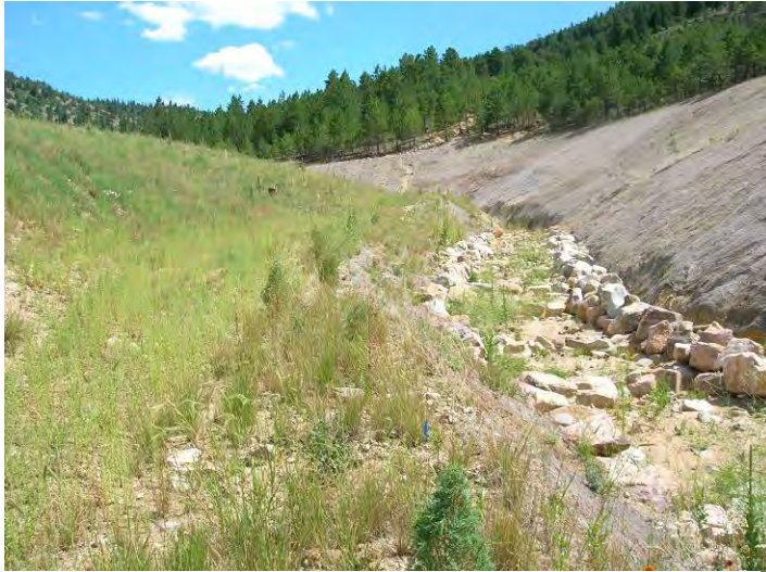
Photo 9. Balarat Gulch Diversion Channel, 2006.
