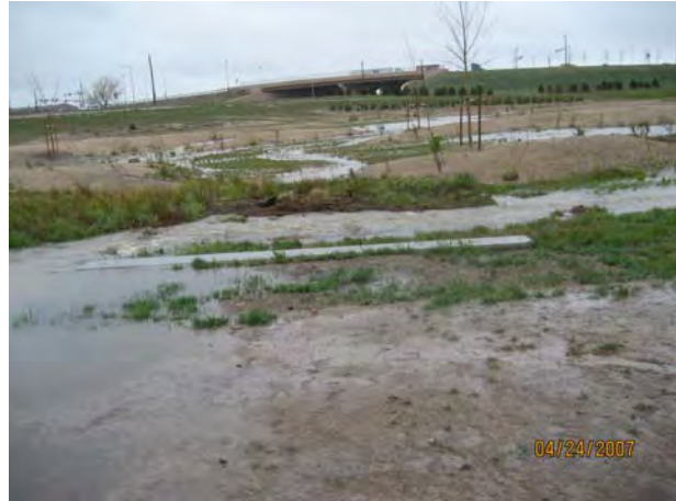
Figure 16 – View looking west northwest at the cut-off wall between Cells 2 and 3
