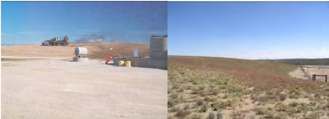
Shell hydro-seeding with Shell seed mixture: December 2005 (left) and October 2007 (right).
