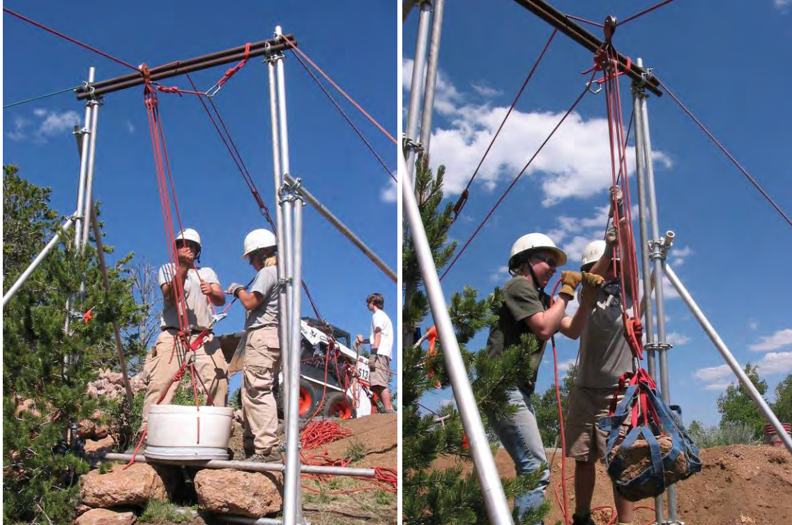
Figure 1 and 2. Example of Rock Tram with bucket and rock sling
