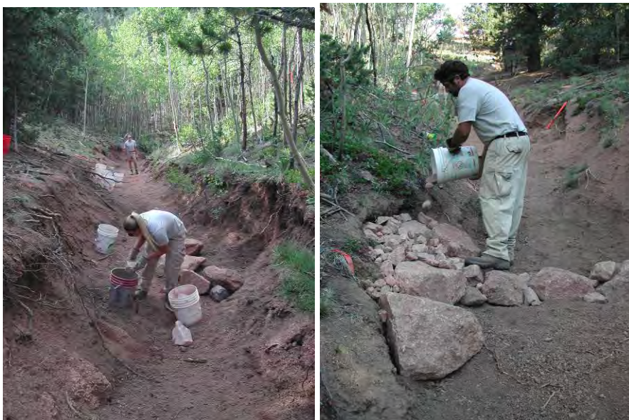
Figure 5 and 6. Examples of building the check dams.
