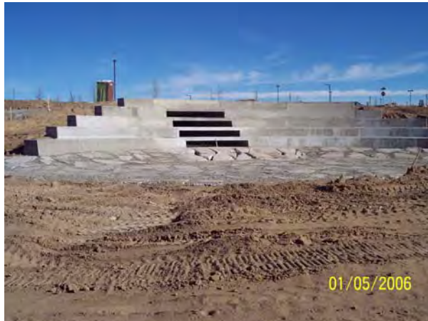
Figure 3-7' x11' outfall structure
