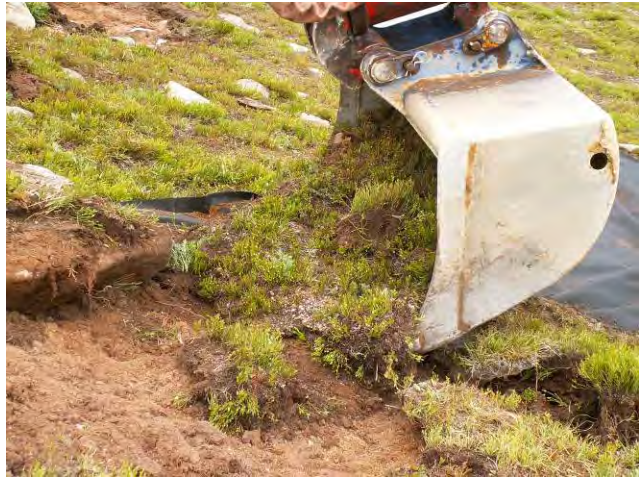
Photo: Welded bar for topsoil salvage spider hoe machine plant and topsoil salvage together
