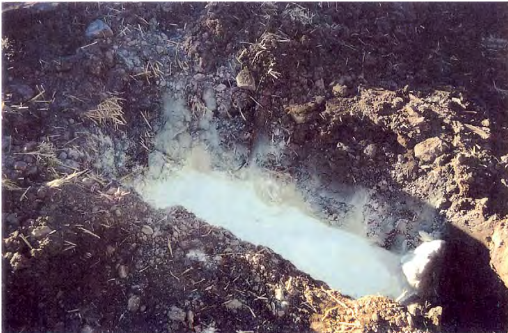
Photo 10. Clay dike in drainage ditch.
