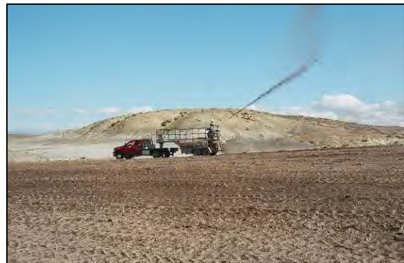
Figure 4. Hydroseeding Warbonnet 11-10 site 10/5/04.
