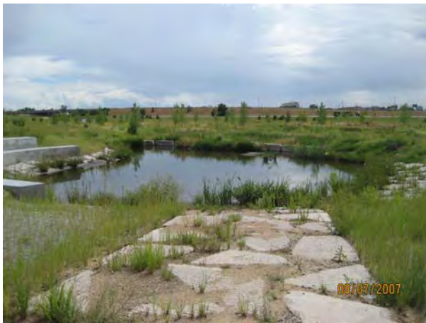
Figure 19 – View looking east at the access drive in the 66" forebay
