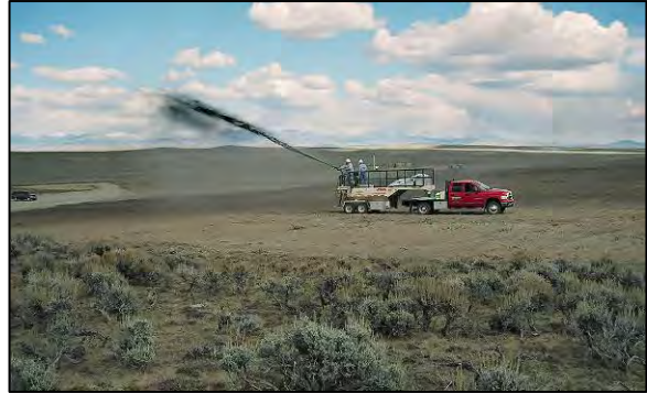
Figure 5. Hydroseeding Antelope 2-9 site 10/4/04.
