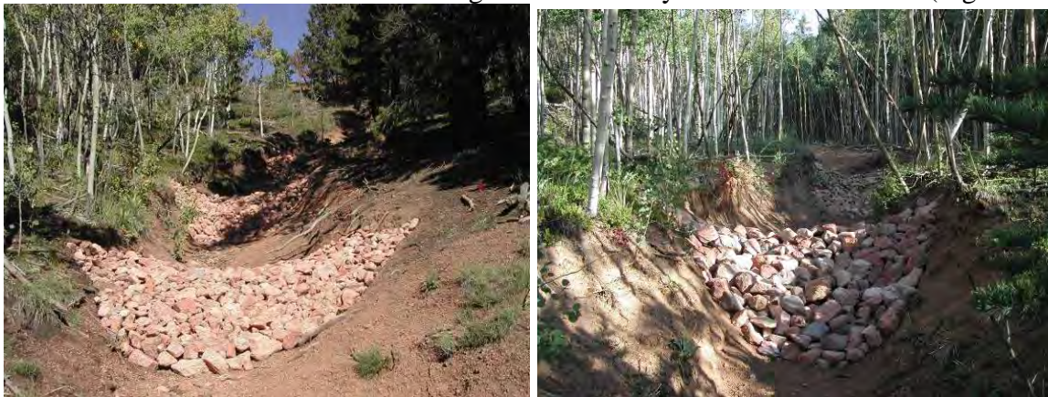
Figure 7 and 8. Examples of finished check dams.
