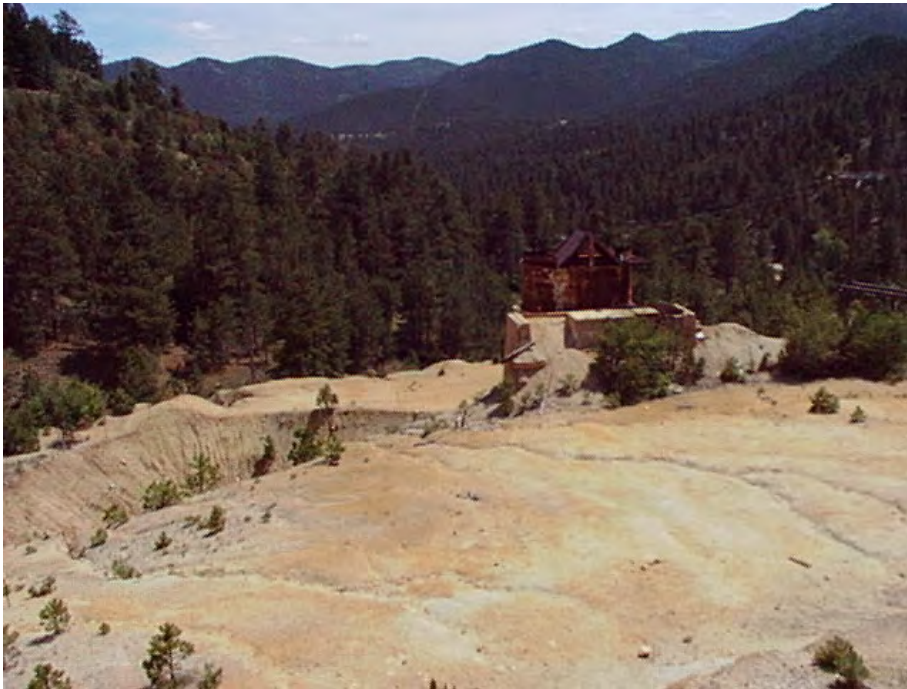
Photo 2. Ore bin and loading structure amidst waste unvegetated waste rock pile.
