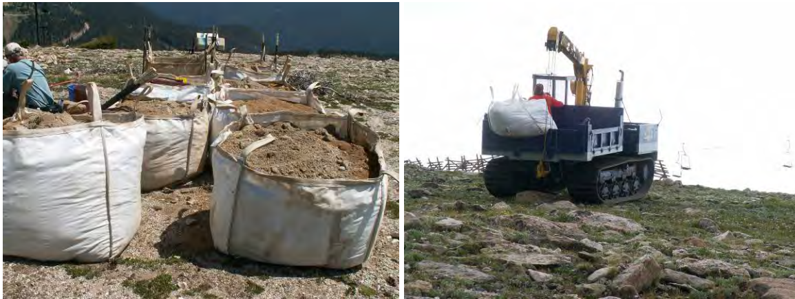
Photo: Soil bags used above treeline. Limited loose soil on undisturbed ground. (Right) One soil bag was removed by Maruka rubber tracked dump truck the others were removed by helicopter
