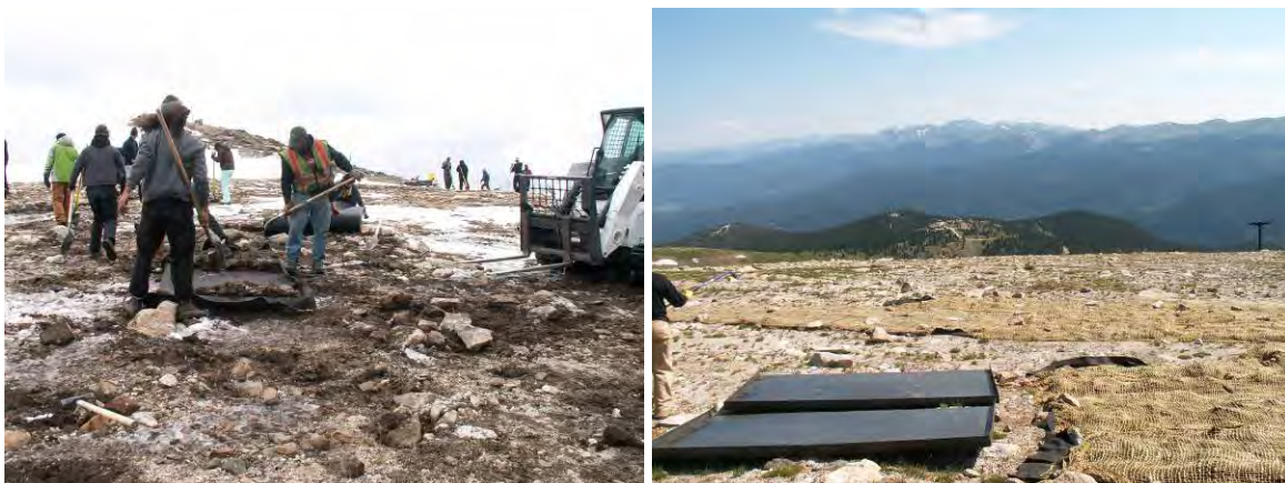
Photo: Panoramic lift (12,000), hand plant salvage placed on tray, picked up by bobcat and set outside disturbance area. Plant material is covered in jute mat.
