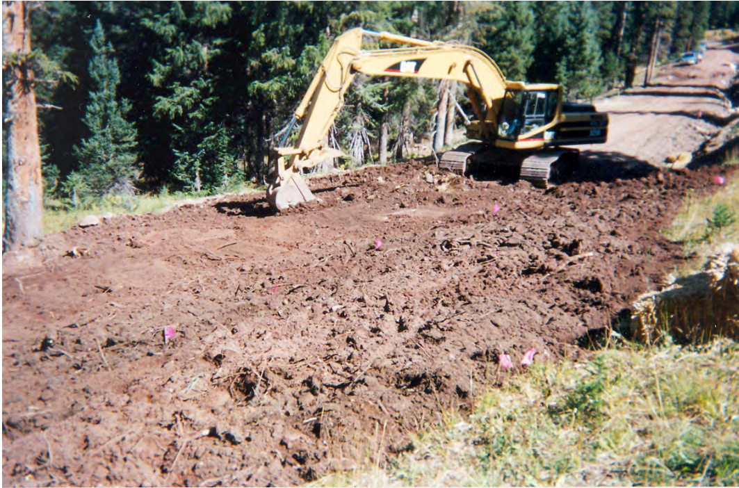
Photo 7. Trackhoe used for restoring wetlands.
