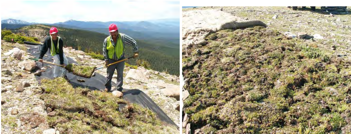
Photo: Eagle Wind (11,500') plant salvage large sections. Placed on geotextile outside disturbance
