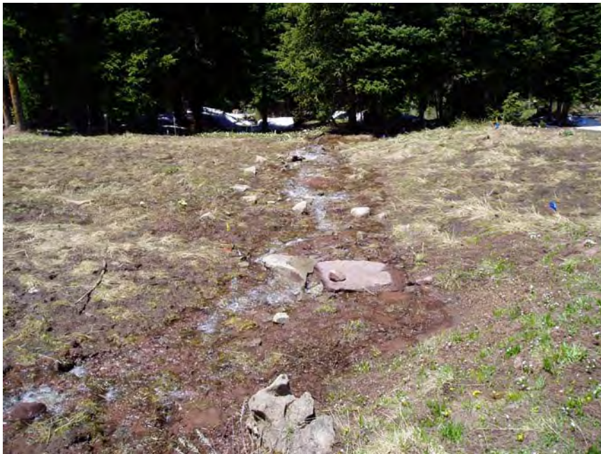
Photo 13. Restored drainage in Wetland 6, June 2007
