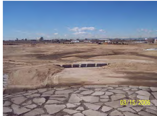
Figure 4-South view of grading
