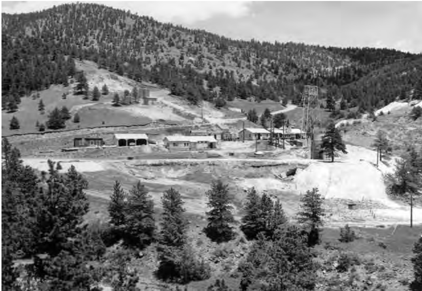
Photo 1. View of the Burlington fluor spar mine complex, around 1940, including the mine adit, waste rock pile, residences and a hoisting tower.
