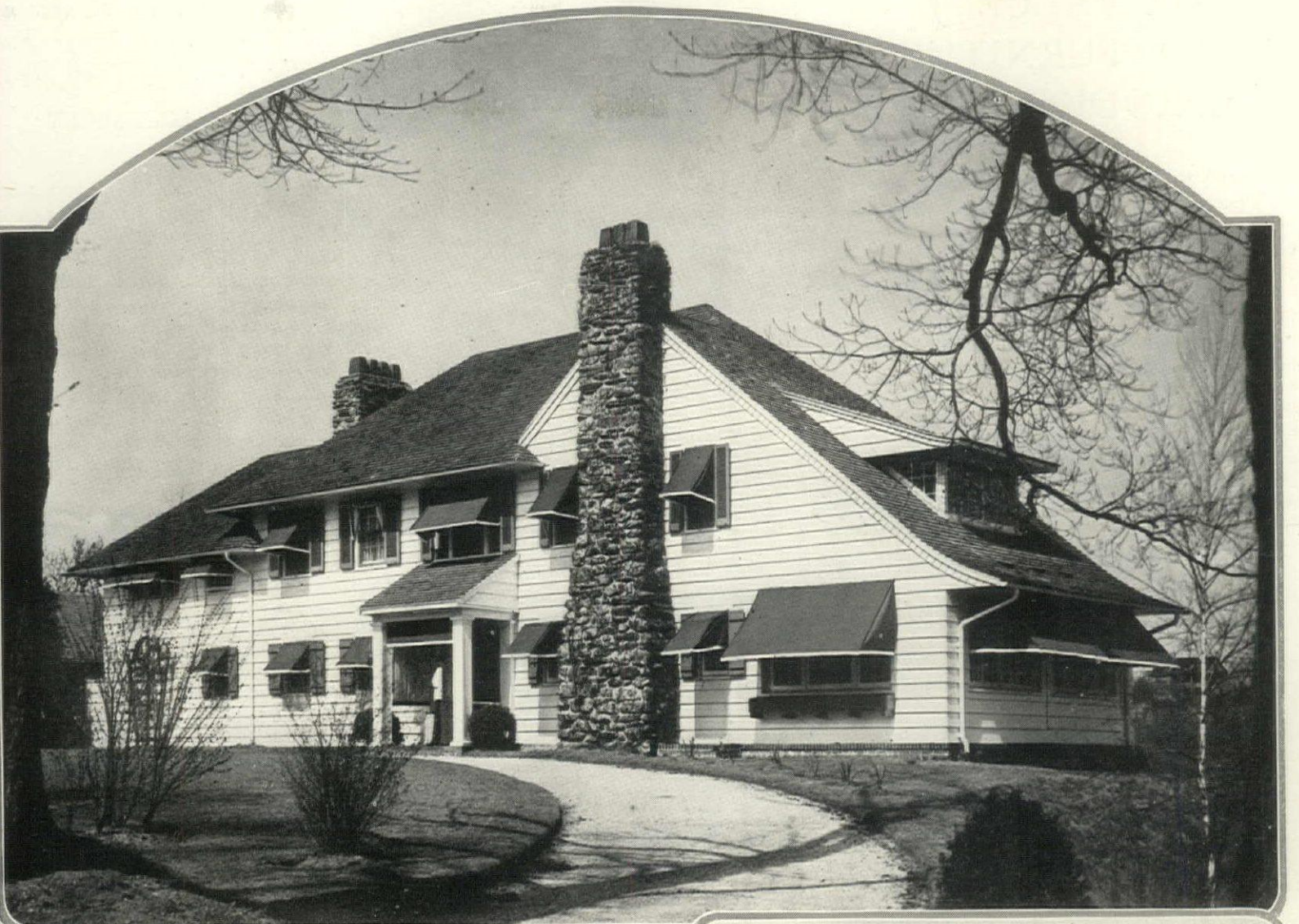
Gillies The house, a reproduction of one in Sussex, stands on the Tom Paine estate. It is white clapboard with green shingles and blinds. Half awnings are in field green and white. A rough chimney adds contrast
