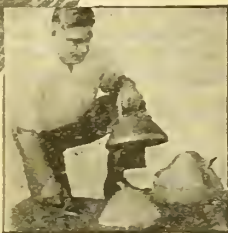
4. Tamp Soil Around Edge of Setter.
