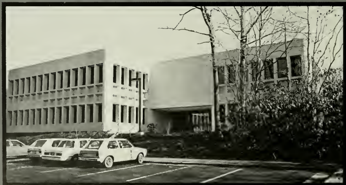
The newly erected University Hall houses the Con Ed Division.
