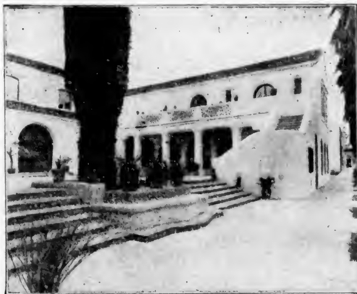
The approach from El Molino avenue, showing giant palm in the foreground, a landmark preserved and around which the project was grouped.
