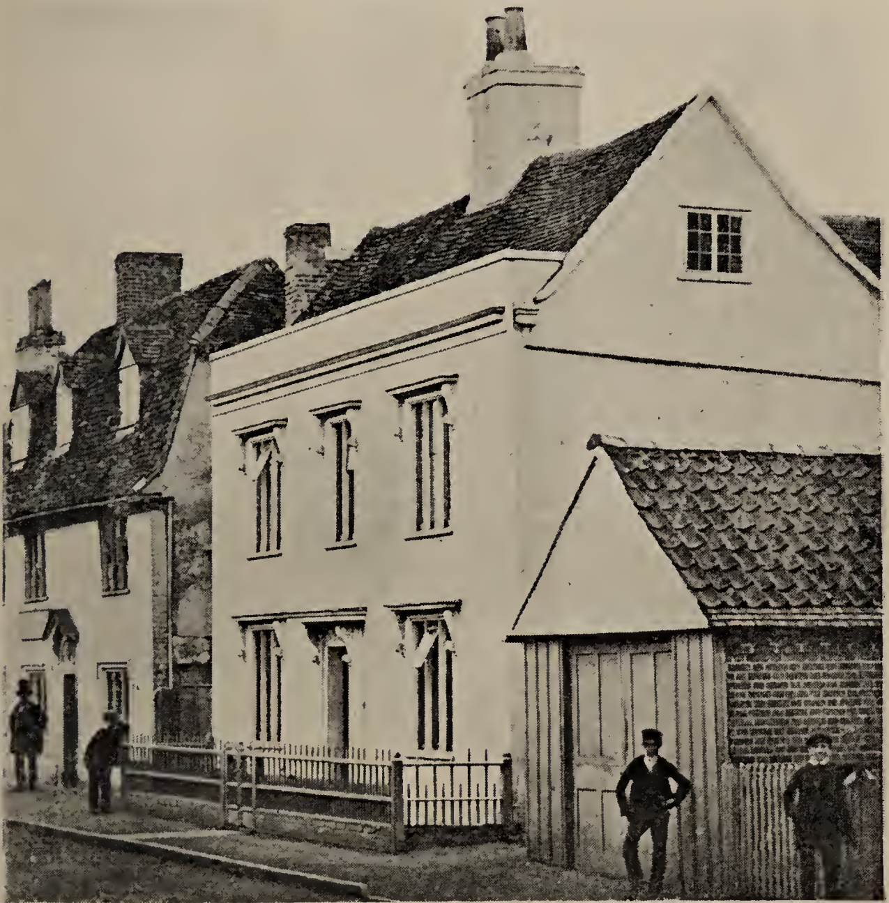
FIG. 2.—HOUSE IN THE HIGH STREET AT KELVEDON, INHABITED FOR MANY YEARS BY E. G. VARENNE (1811-1887), BOTANIST.
