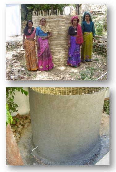
Fig 5.2.6.1 and Fig. 5.2.6.2 Bamboo-cement based rain water storage tank under construction
