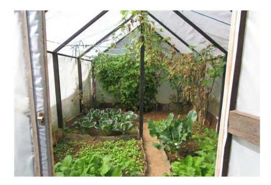
**Greenhouse:** Traditional greenhouses can be expensive to construct and the materials aren't always easy to procure in remote areas. Therefore, the design being adopted for the EVD programme is a low-cost model that is constructed out of a bamboo or wooden frame and ultraviolet-stabilized plastic. These closed structures help grow vegetables, herbs, or flowers in off-season times. They also protect plants from being ravaged by animals, birds, and other plant eaters.
