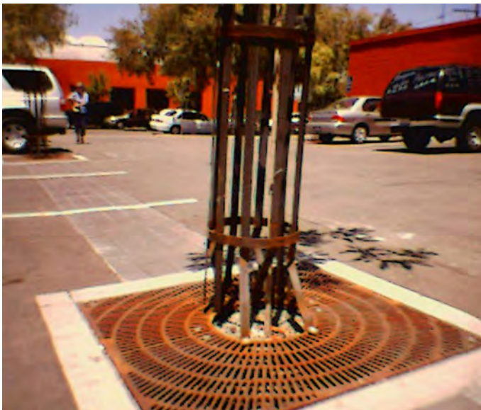
Fig 50: Palo Alto was the first western city to use the Cornell University patented method planting mix (390 Lytton—not shown) and in the above photo, structural soil 24" deep provided room for the roots of this Chinese pistache—below the parking lot surface—at another downtown location.
