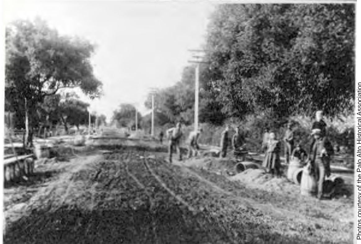
Fig. 1: Professorville streets were already lined with trees when they were paved. Presumably some of these trees were native and some planted by residents. This photo shows paving work being done to the section of Waverley Street between Kingsley and Lincoln circa 1902.
