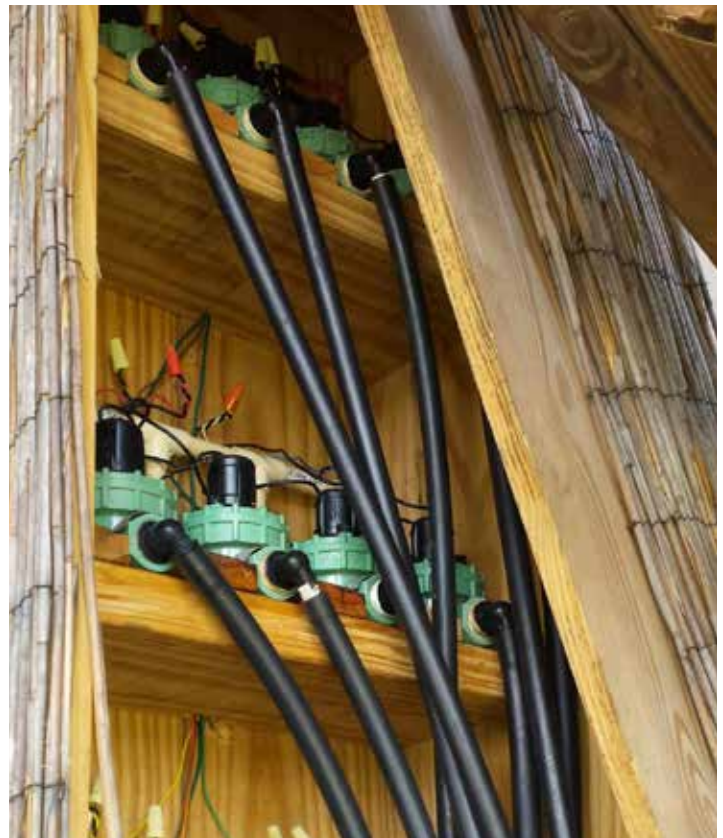
Out of this world circuit breaker
