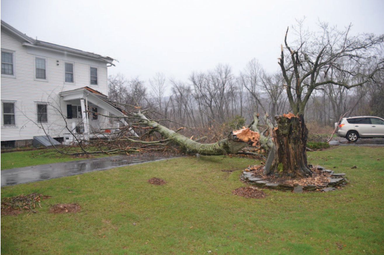
UNADILLA – Around 5 p.m. on Easter Sunday, April 16, a brief but powerful storm with wind and rain passed through the area. Several branches and trees were felled by the high winds, including this large maple that came down on the porch and corner of the Connor residence located on Main Street, near Wattle’s Ferry. In addition to structural damage to the home, one of the oldest in the village, a few of the Connors’ vehicles sustained damage from falling limbs. Photo credit: Anna Ritchey.
