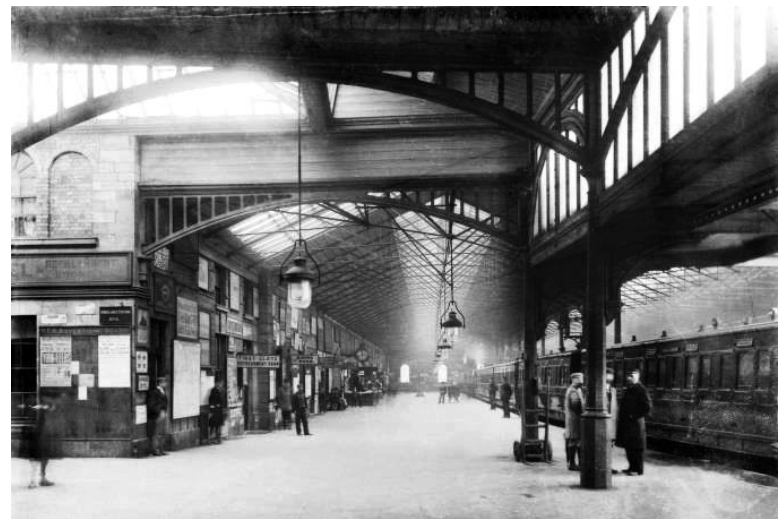
Right: Inside Scarborough station in 1898 looking down the end of the platform showing ornate gas lighting. The wrought iron and glazed roof can be seen in the photo. On the left side are waiting rooms and the clock in the far distance is above the entrance and exit
