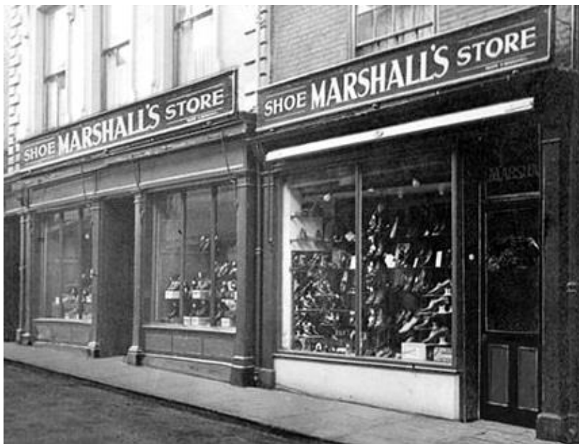
Above: The shop in the 1940s when it was called Marshall's Shoe Store.
