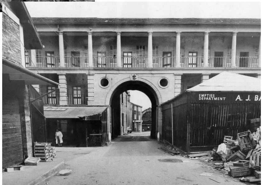
Right: Looking through the South Gate entrance towards Horton Street from inside the wholesale market at the Piece Hall before the cantilever bridge was replaced with an electrically powered lift bridge. On the left is part of one of the buildings that were built in the centre of the courtyard with a lean-to and the shed on both sides of the entrance.
