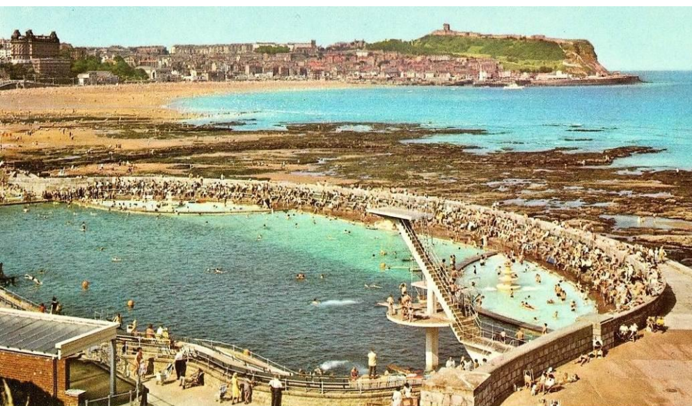
Left: The South Bay Pool with the 32 foot high diving board illustrated in Oakdale's poster of 1936, but with additions made in about 1950. After being modernised in 1934 it has two semi-circular shallow pools for children with fountains, a walkway around the sea-facing side of the pool and the sea walls were increased in height allowing for additional spectator seating. Its popularity is shown by crowds sitting on the wall around the pool
