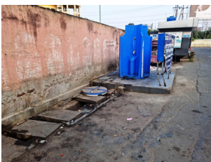
Figure D: unhygienic surroundings of Public Toilet
