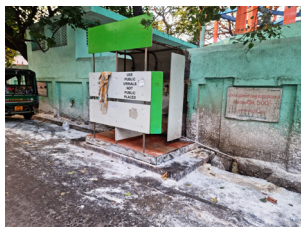
Figure A: unhygienic surroundings of Public Toilet
