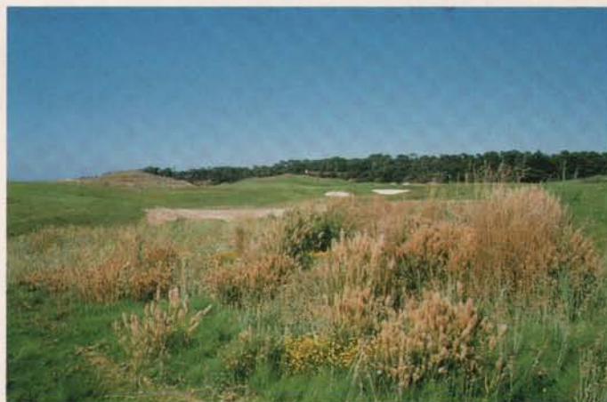
The same hole following construction accented with dune grasses.
