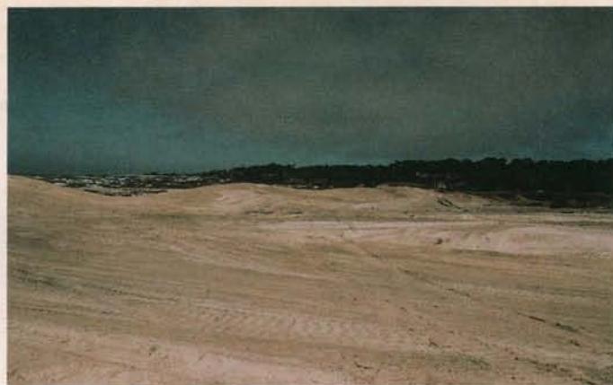
The 18th hole prior to construction.
